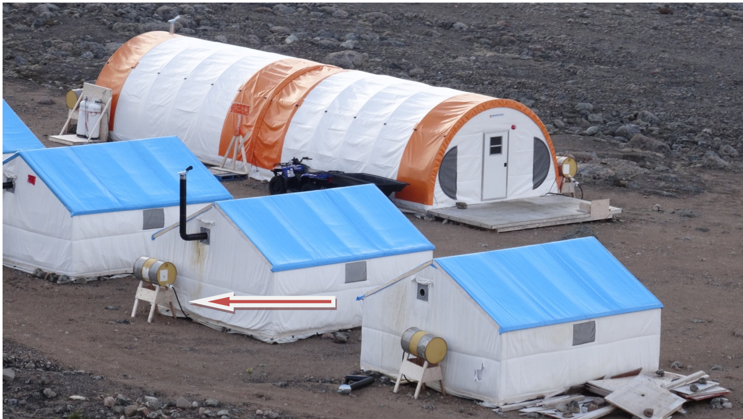
Photo 3: Drums behind tents used for heating fuel tanks not in secondary containment. Arrow identifying wooden fuel stand.
