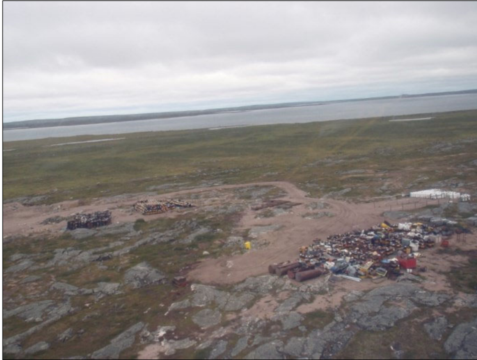
Photo 1: Fergusson Lake Camp waste pile prior to initiation of remediation work.
