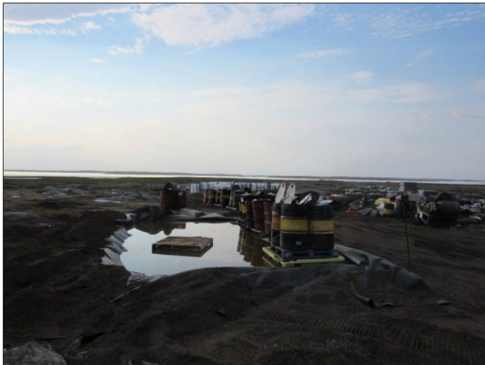
Photo 2: Temporary lined berm for containment of waters from waste drums.
