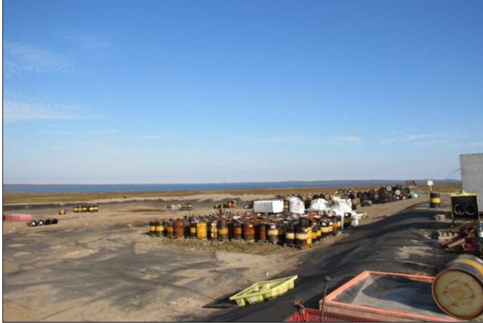
Photo 5: Main lined berm containing excess, now dry, waste-filled drums.
