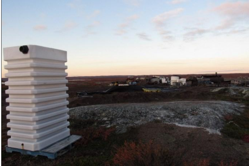
Photo 3: Plastic tank used for containment of excess waters from berm.
