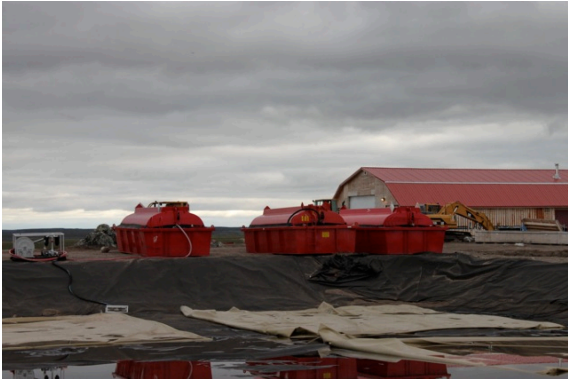
Three Enviro Tanks - double walled tanks
