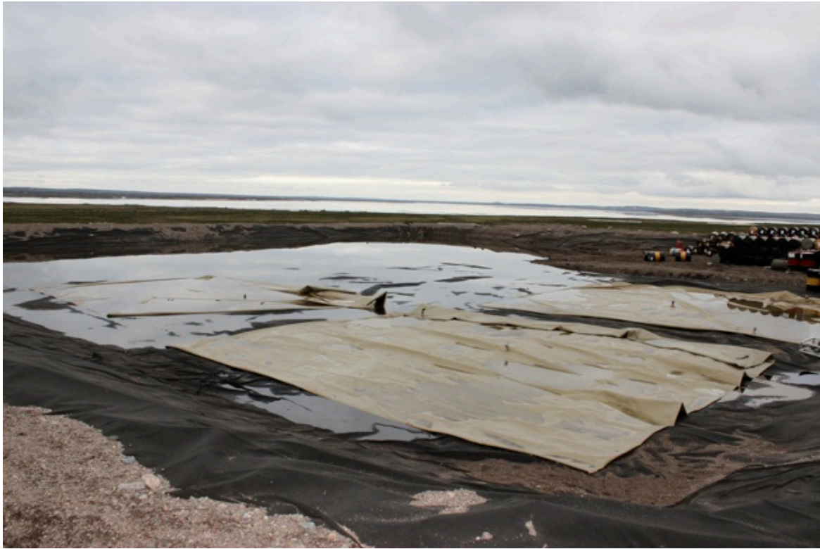
Lined Earthen Berm - all three fuel bladders remain empty
