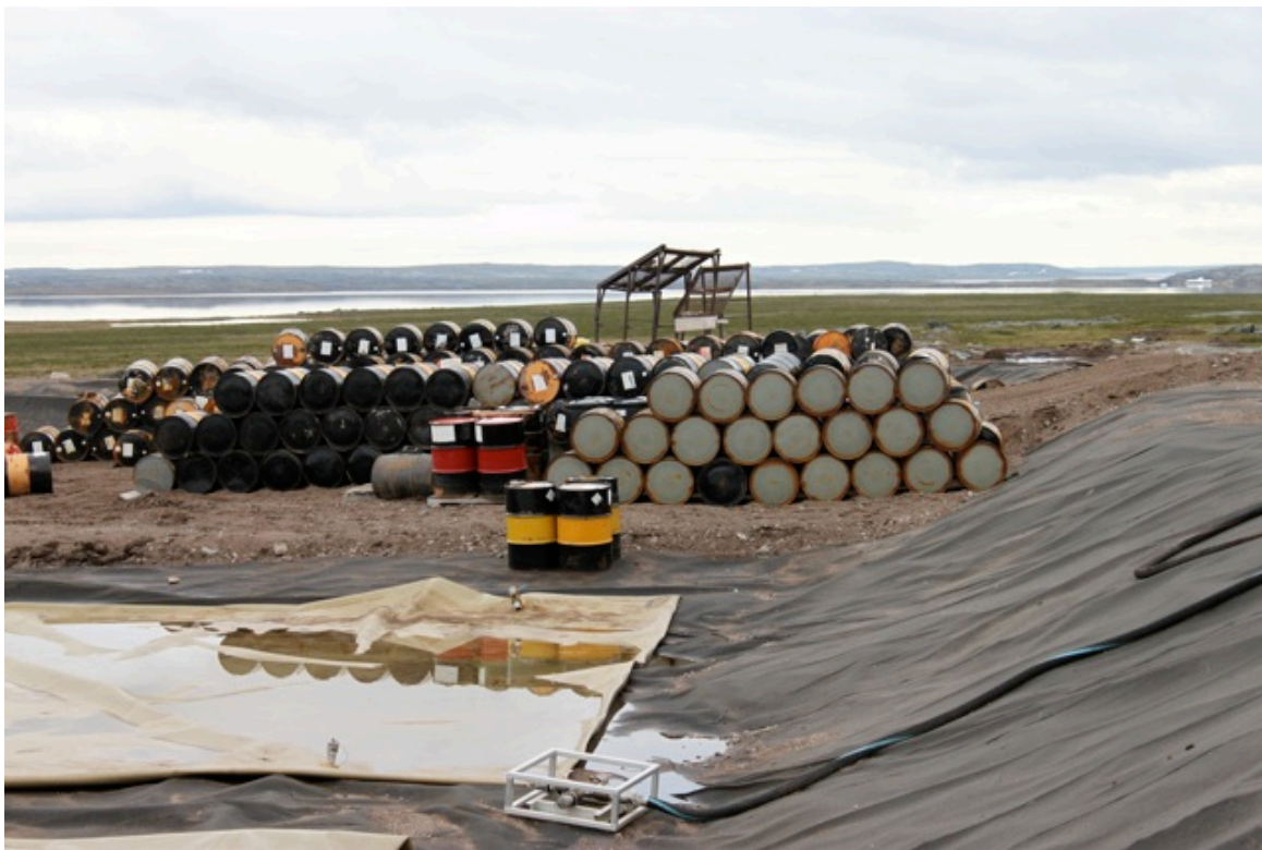
Drummed Fuel - stored in neat rows within the lined earthen berm
