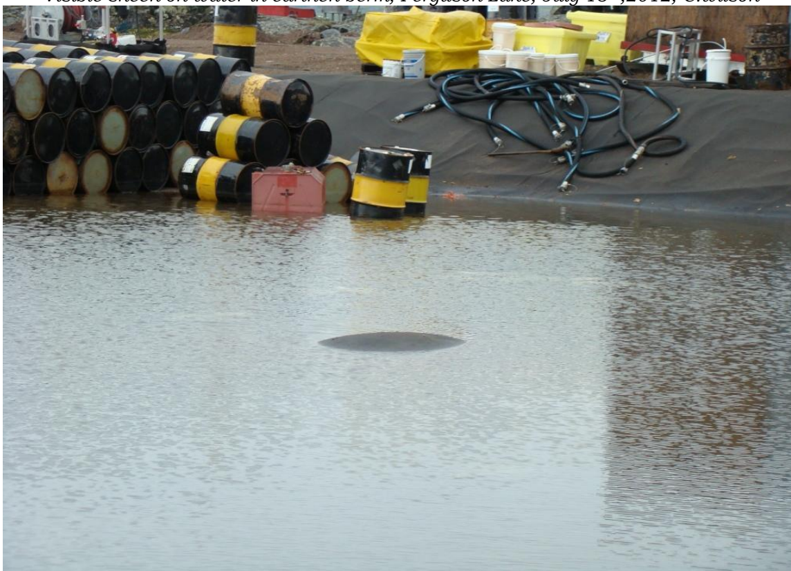
Bubbling in impermeable liner, earthen berm, Ferguson Lake Camp, July 13 th , 2012 C.wilson.
