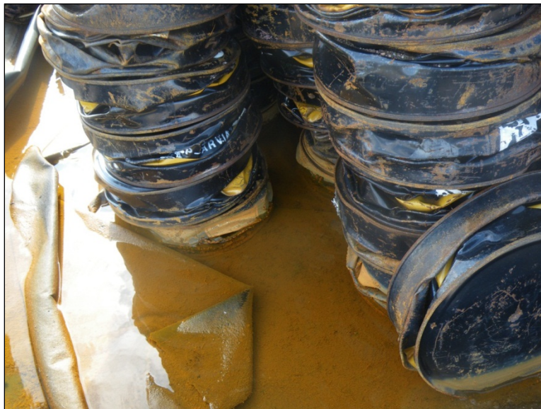
Plate 6. Standing water in crushed fuel barrels berm with amber colour and visible oil sheen.
