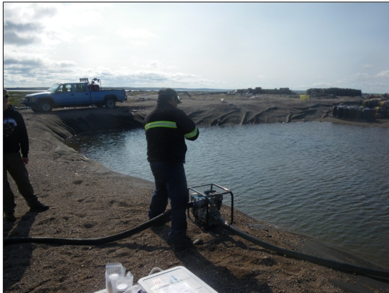
Plate 4. Maintenance worker setting up pump at the centre of the northern edge of the fuel berm area.
