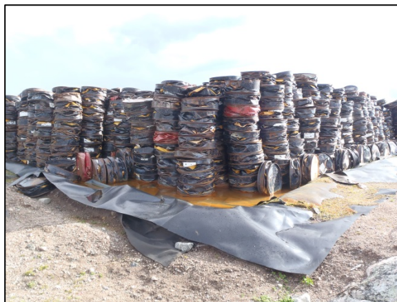
Crushed drum berm
