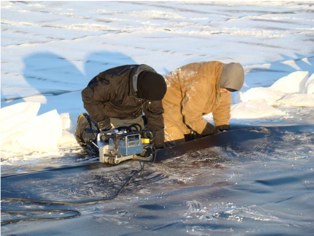
Welding the liner of the secondary containment storage area.
