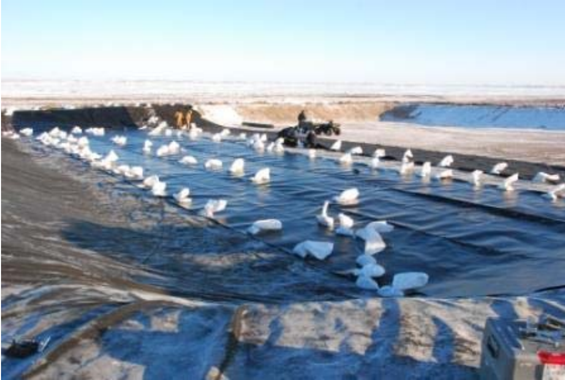
Lined-bermed secondary containment storage area for fuel.
