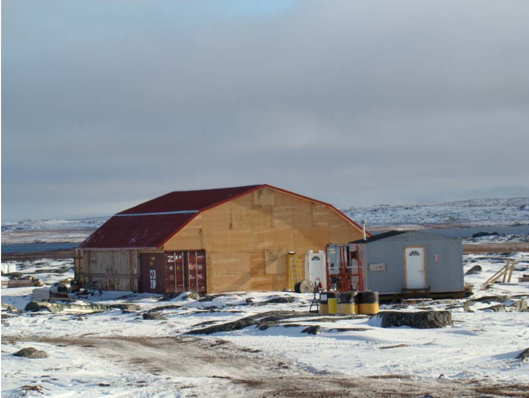
Workshop constructed using two seacans.
