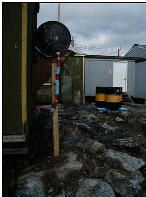
Plate 2.1-6 Typical view of fuel tank mounted outside of huts (Hut 7).
