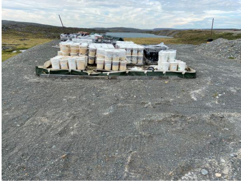
Figure 1. Contaminated material adjacent to berm has been remediated and material spilled material has been removed from the berm.
