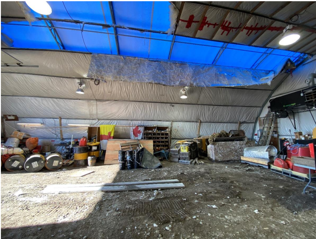
Figure 3. Quonset after high risk insulation removed and showing no ponding water.
