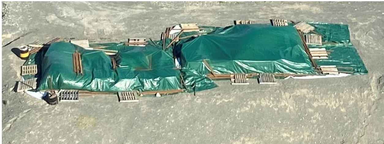
Figure 2. Pop-up berms covered completely with tarps.
