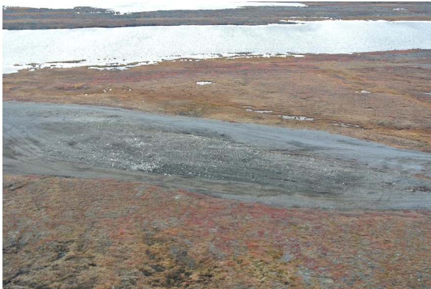
Post-reclamation Cuttings Sump
