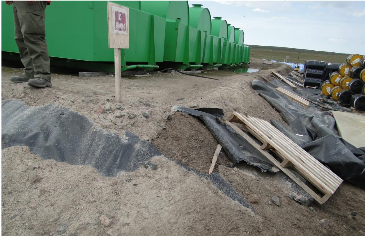
Figure 15. Torn liner for bulk fuel storage.
