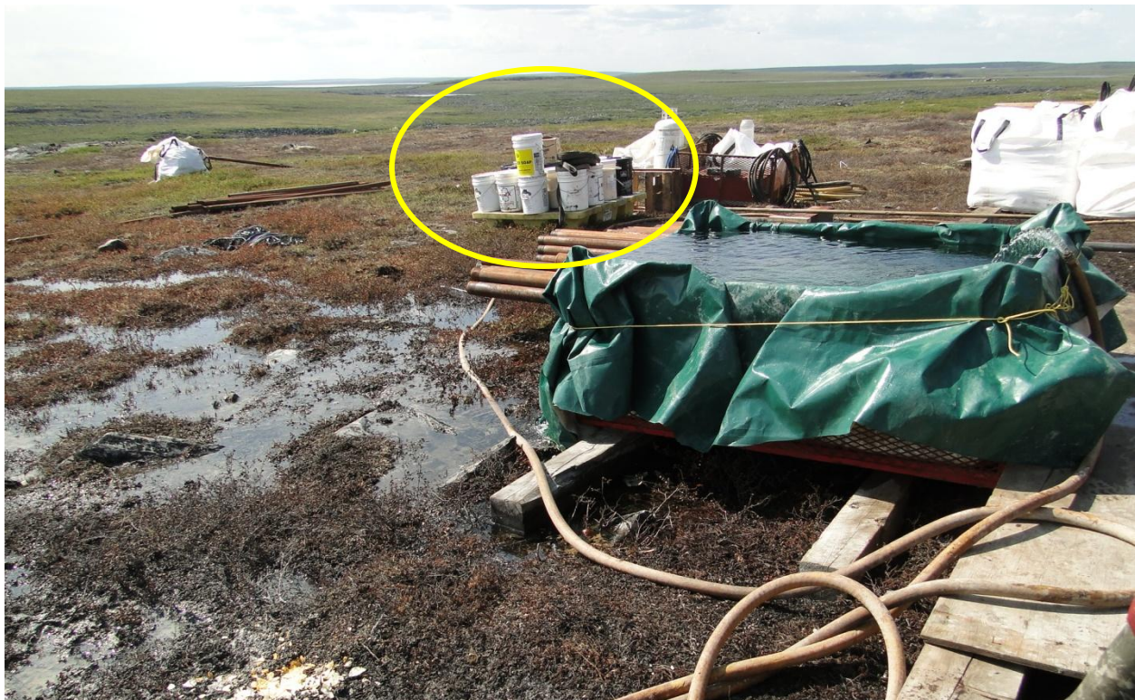
Figure 16. While technically 'on' secondary containment, the efficacy is doubtful.
