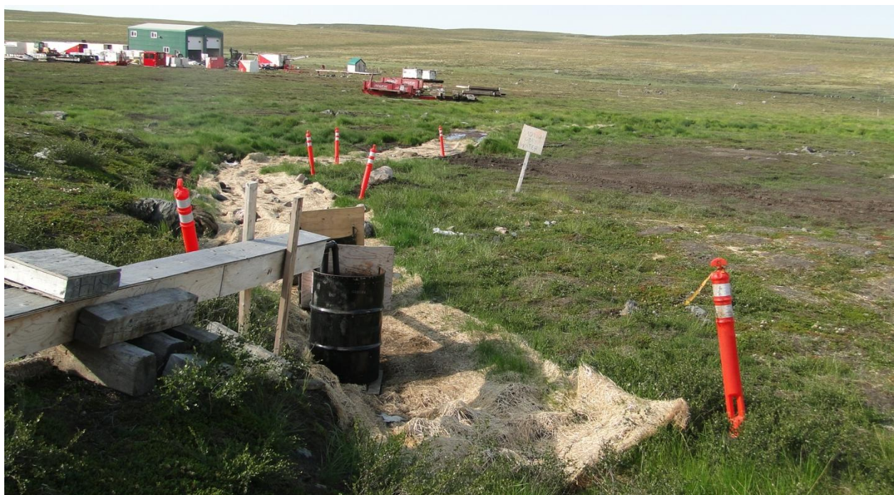
Figure 6. Grey water discharge - improvised grease traps and fibre matting to settle particles out. No defined depression to act as a sump.
