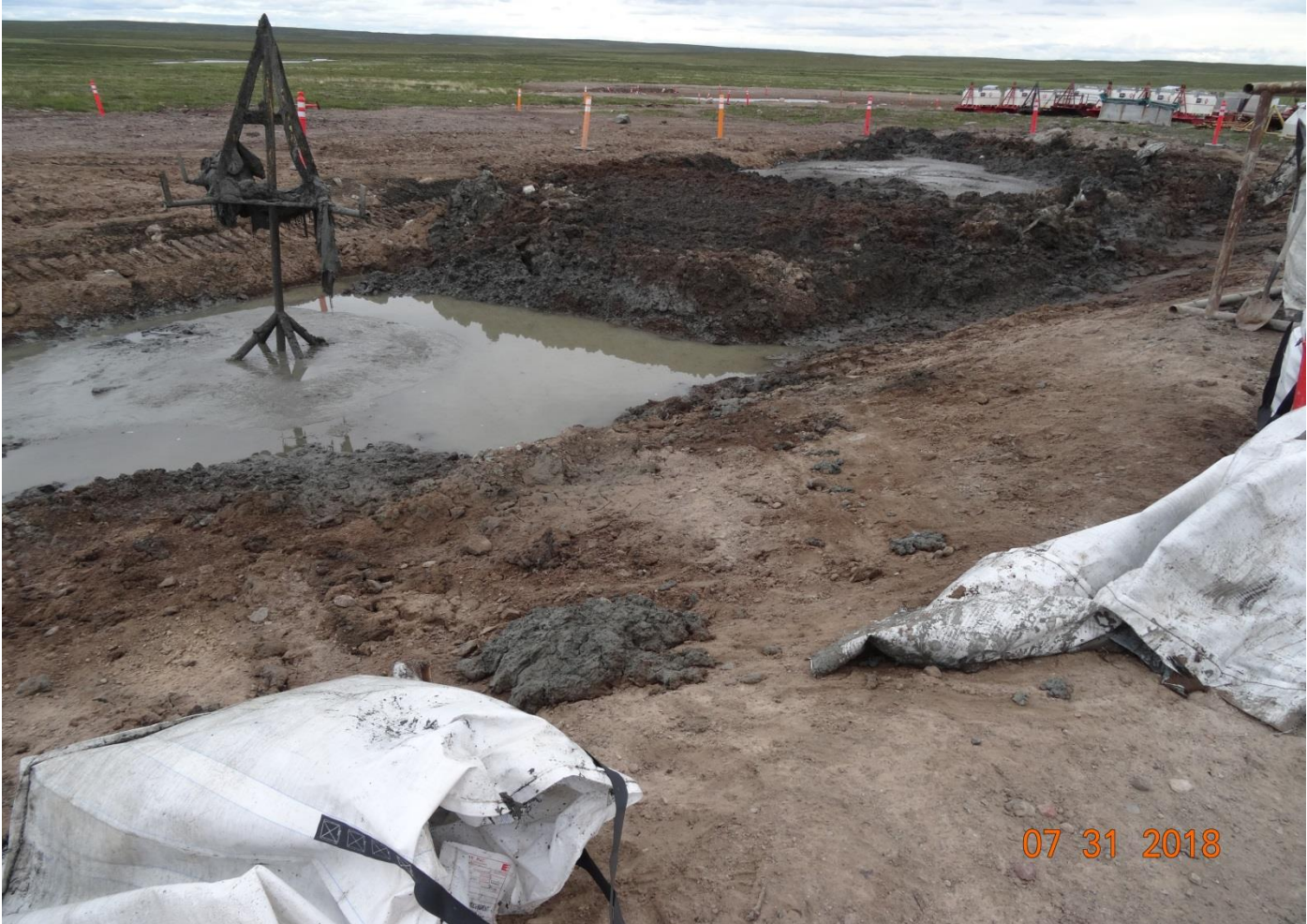
Description: Drill cuttings sump located east of Goose camp
