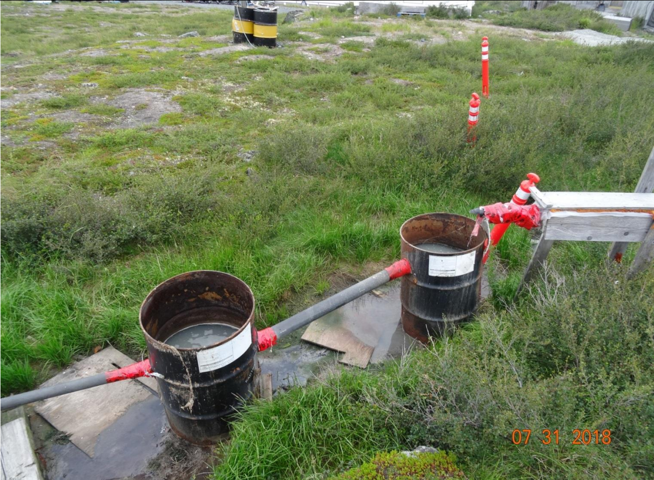
Description: Grey water catchment basins from camp kitchen and main dry
