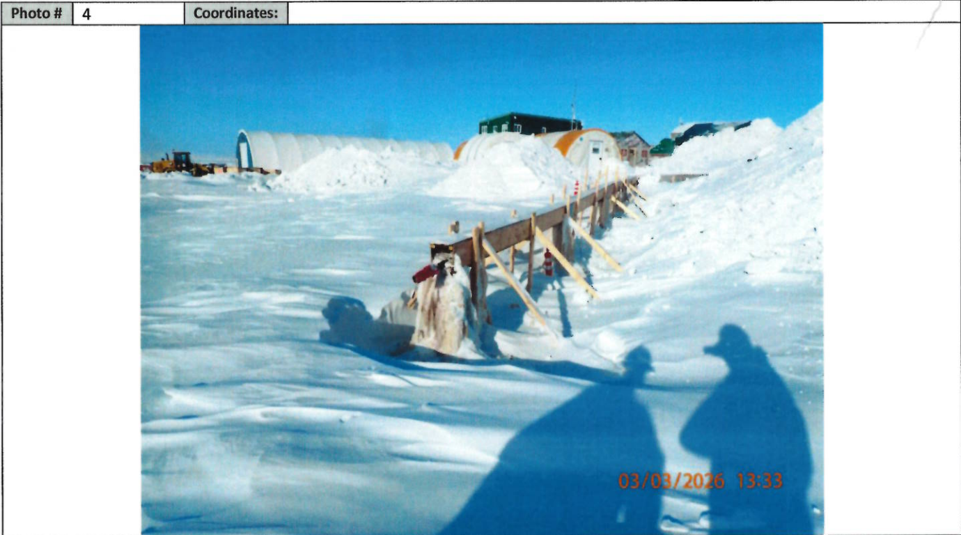
Description: South side grey water discharge location at exploration camp. No signage.
