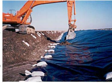
highly UV stabilized flexible liner, that provides the same exposed service life at 30 mil as can be expected from 60 mi
