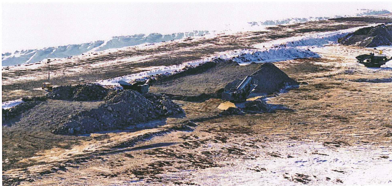
Plate 4. Work in Progress on Airstrip, Showing Crusher and Stockpiles.
