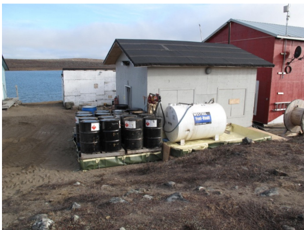
Figure 1: Bulk fuel tank, fuel transfer pump and drummed fuel at main generator, Hackett River Camp. (09/23/2012)
