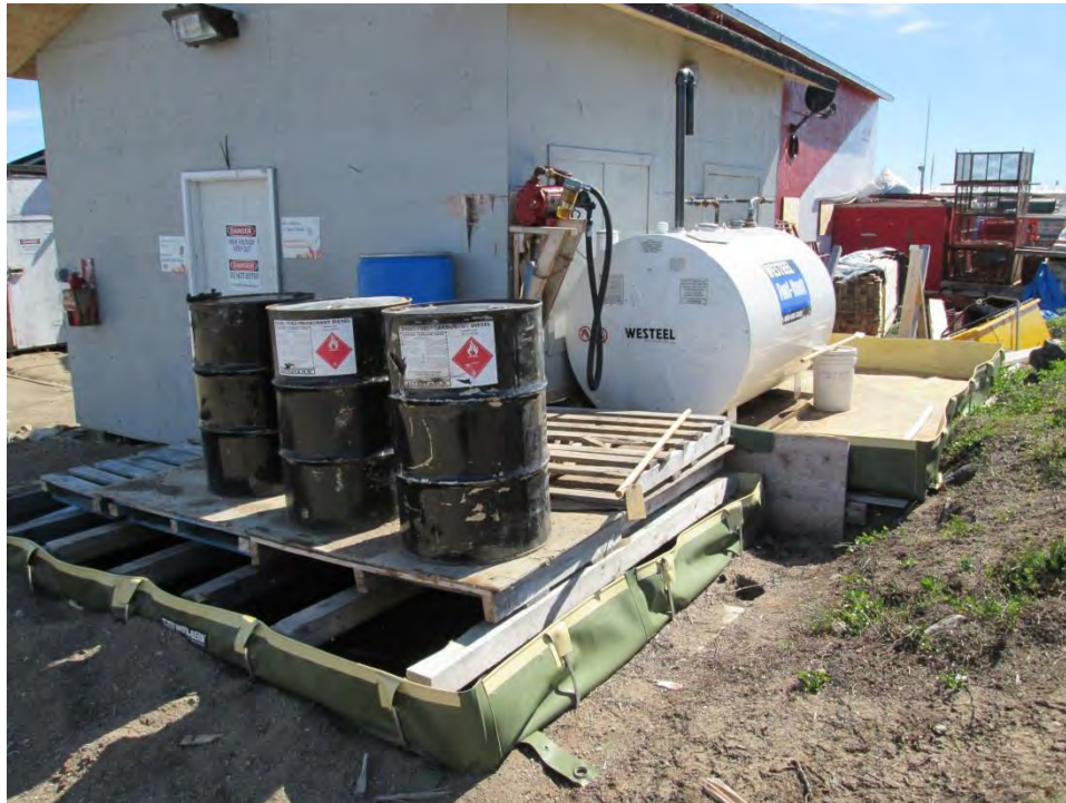
Plate 2: Bulk fuel tank, fuel transfer pump and drummed fuel at main generator, Hackett River Camp. (07/04/2014)
