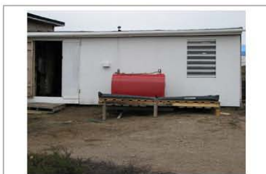
Main Generator fuel tank, and berm.jpg
