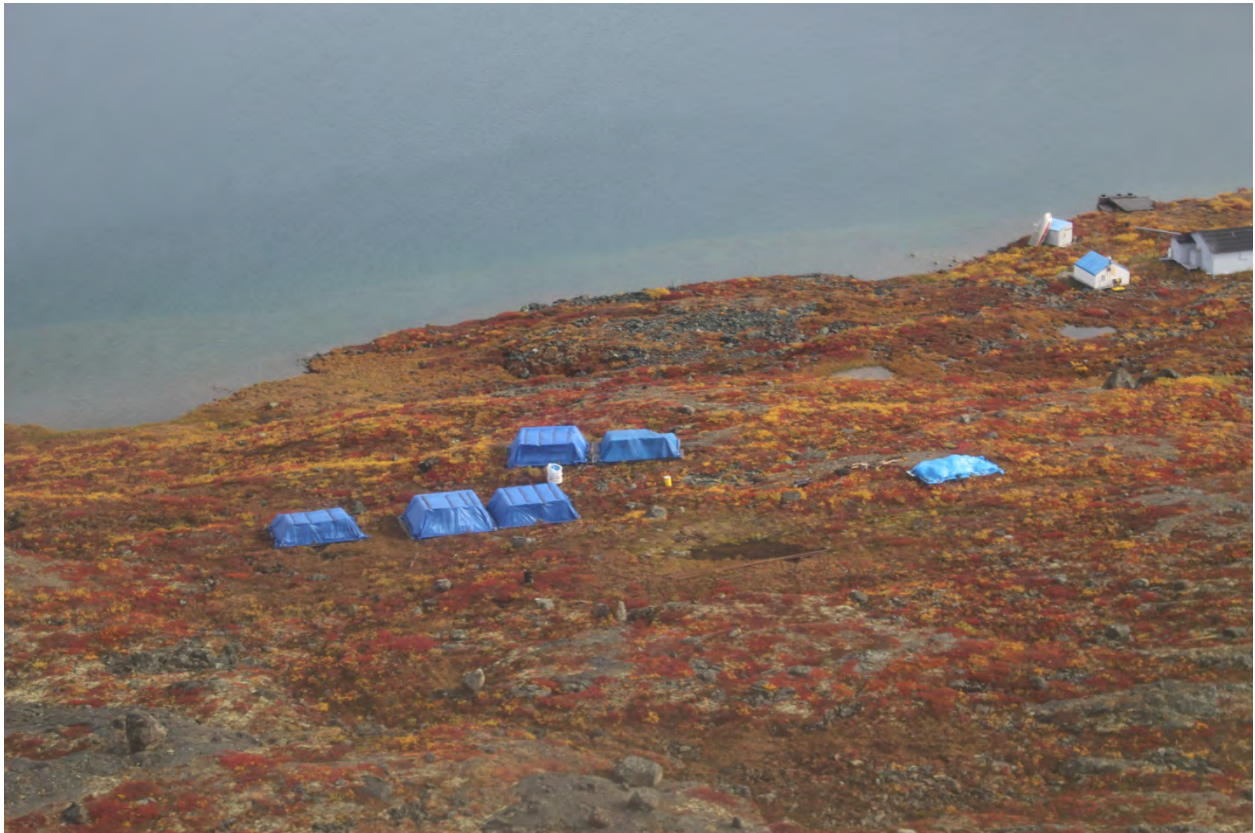
North fuel cache High Lake site showing covered secondary containment
