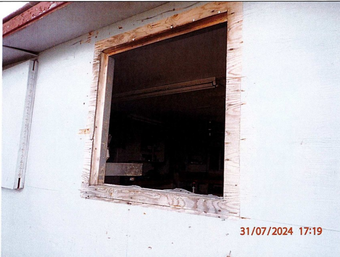
Main building kitchen window open, the plywood was observed on the ground.
