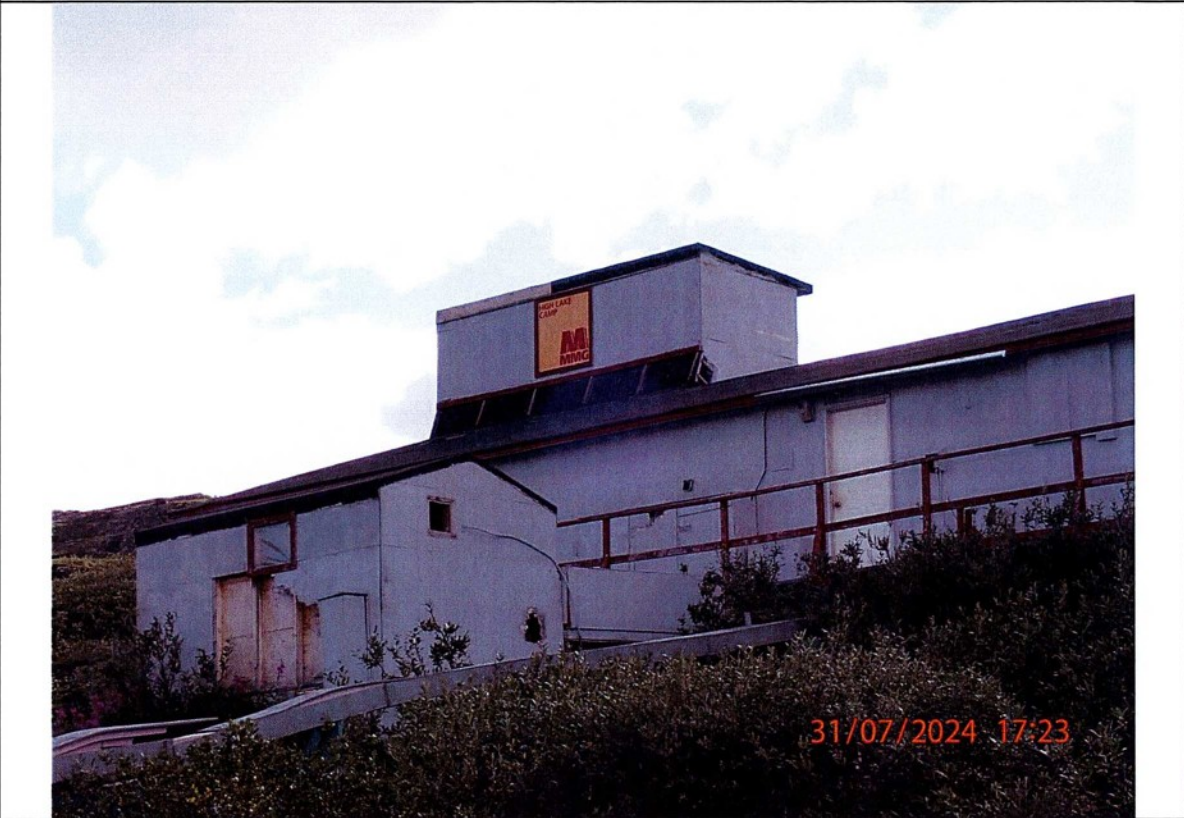
Another view of the shack beside the main building, Plywood from the wall is missing, an open window and a hole in the back wall is shown.
