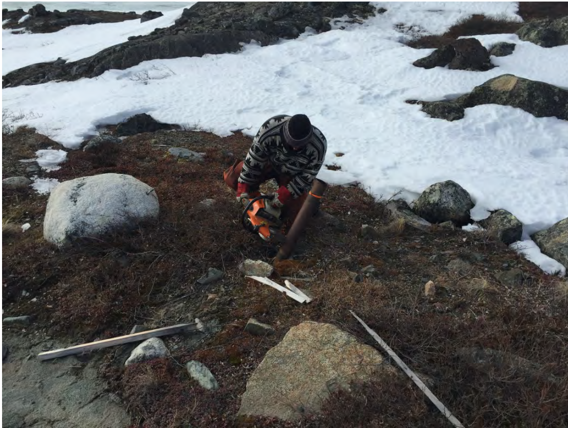
Cutting historic drill casing off at ground level.
