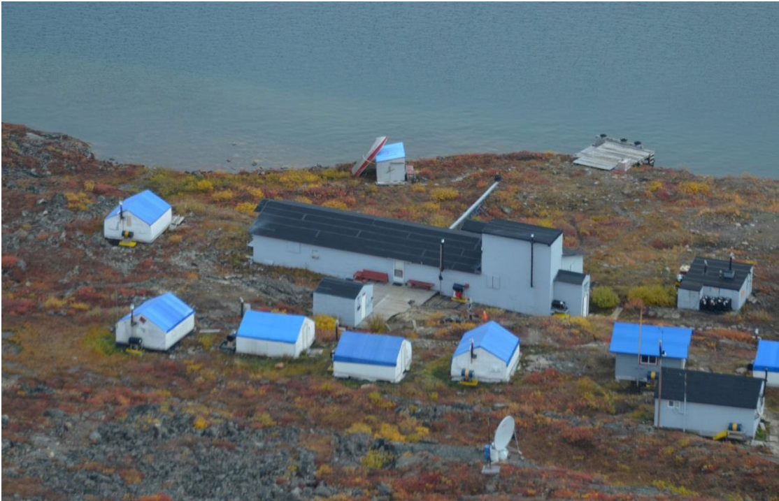
Figure 3 - High Lake Camp site August 2013
