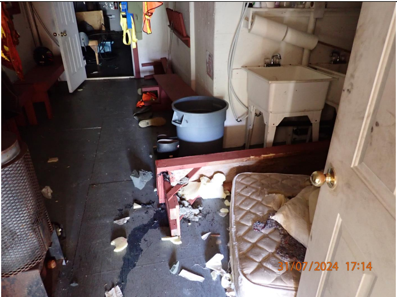
Inside the main building entrance, bear scat is observed on the bench and floor.
