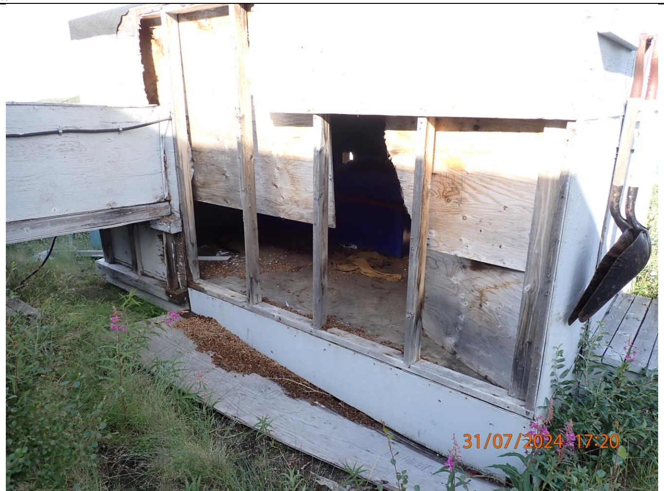
Small shack beside main building shown with an open side wall and ptarmigan droppings inside.
