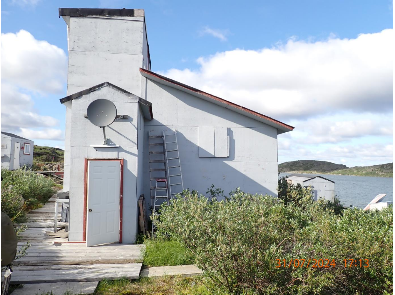
Main building with door open.
