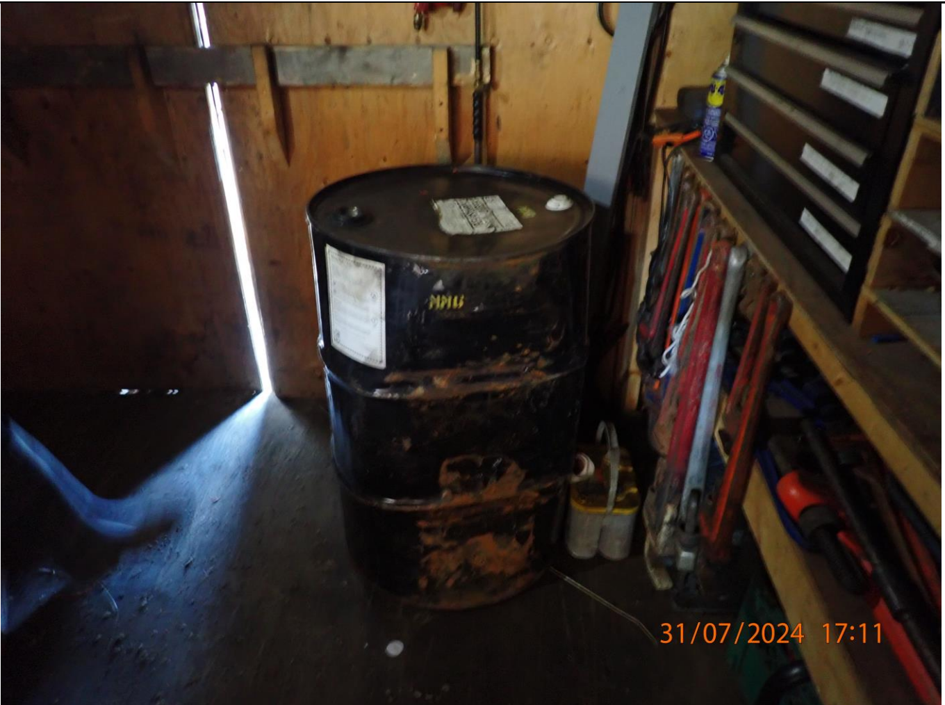
1 fuel drum outside of containment inside the mechanic shop
