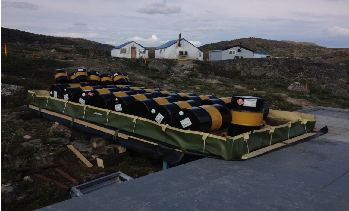
Secondary Containment at Helicopter Pad – High Lake
