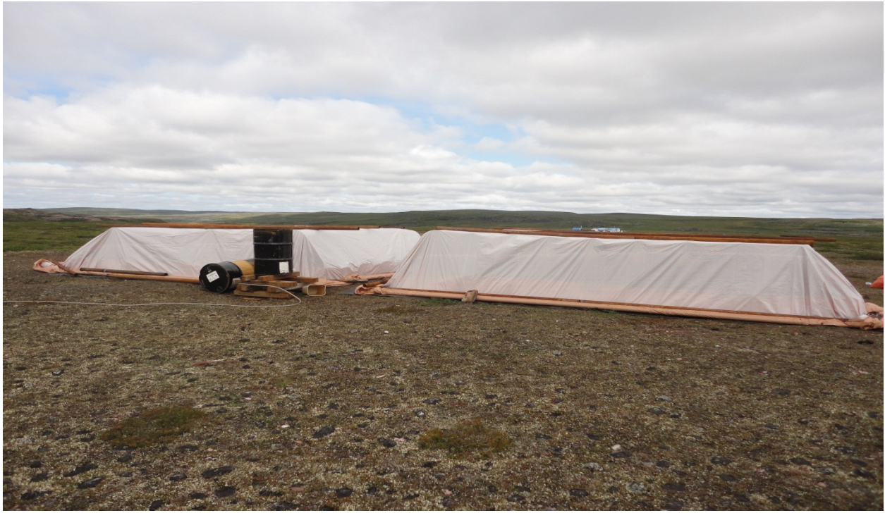
Fuel Cache High Lake East with Secondary Containment and Tarps
