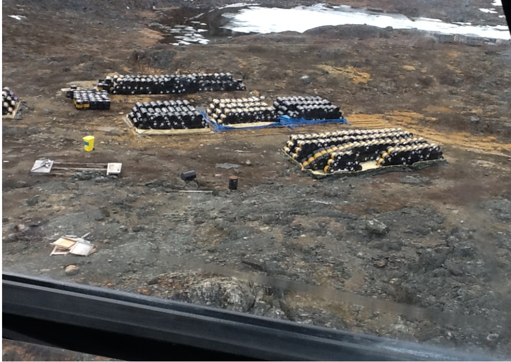
Fuel Storage with Secondary Containment Berms – North Cache High Lake
