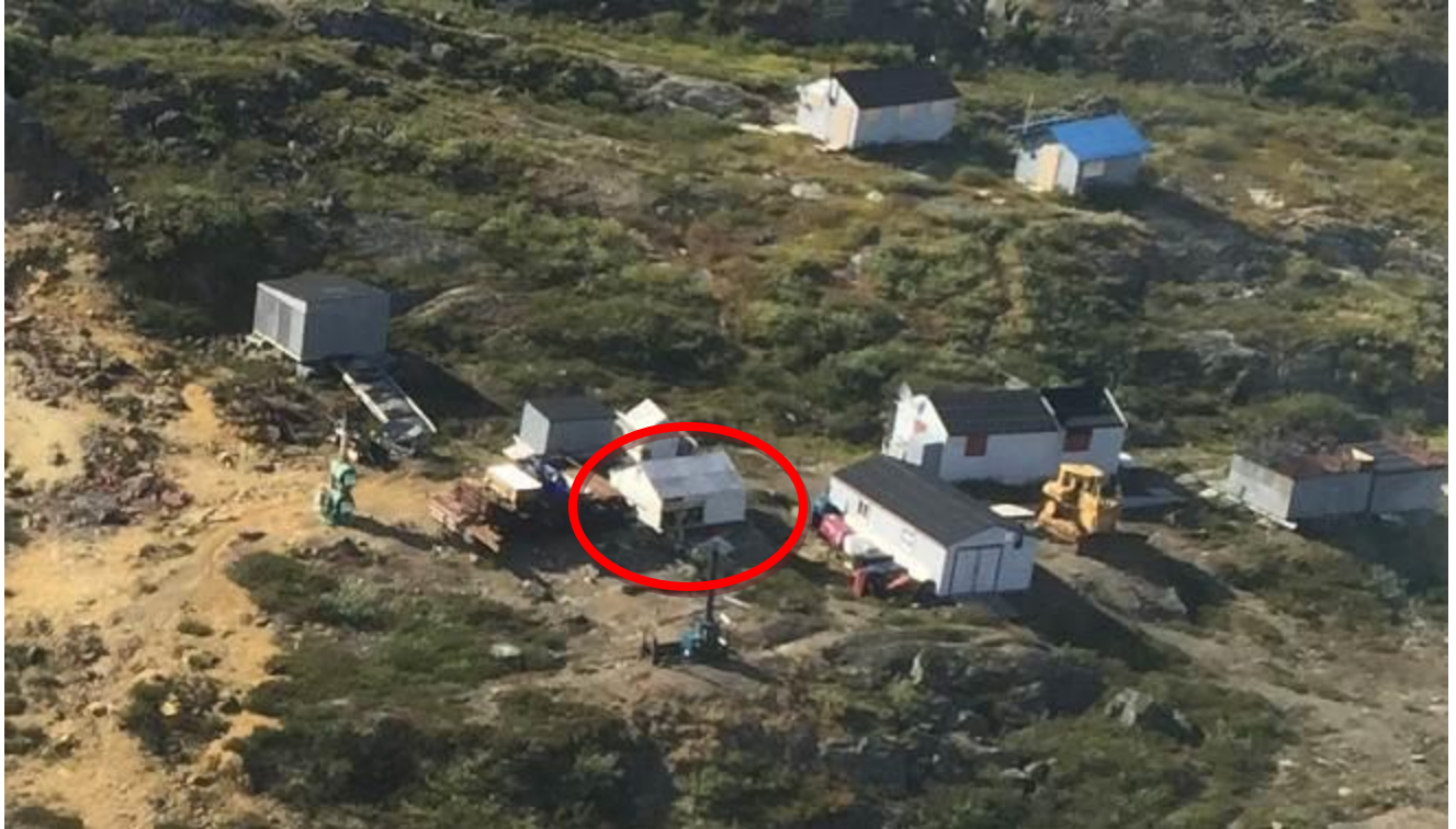
View of High Lake camp looking W. Buildings all appear to be in good condition with the exception of the Coldstore tent which has one side panel that has popped off. The panel will be repaired during the planned 2017 visit.
