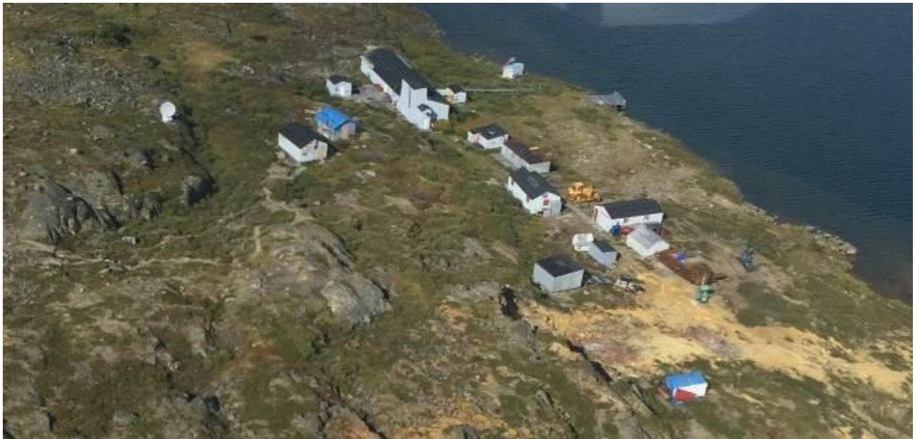
View of High Lake camp looking NE. Buildings all appear to be in good condition.
