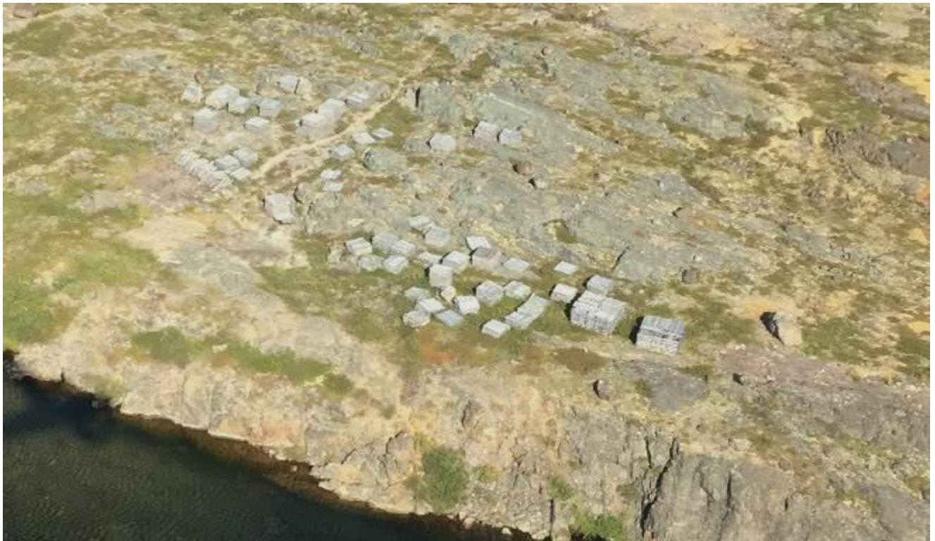
View of "New" core storage area looking E. Racks and core all appear to be in good condition. Core shack building completely removed.
