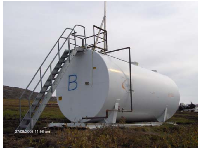
Photo 4 The fuel transferring systems – with three (3) anti-siphoning valves
