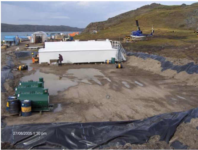
Photo 3 Secondary Containment surrounding 70,000 L AST and the previous Location of spill tank.
