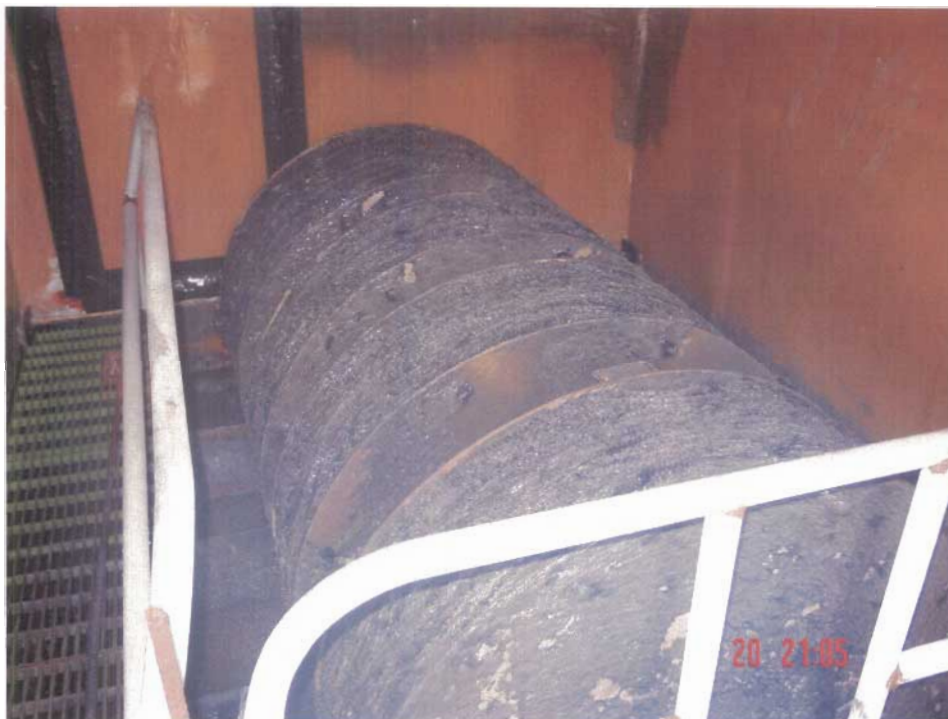
Photo # 4. Interior workings of Rotating Biological Contactor.
