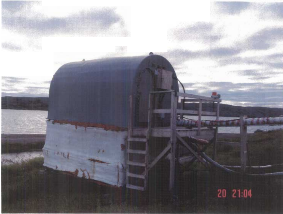
Photo # 3. Sewage treatment system Rotating Biological Contactor.
