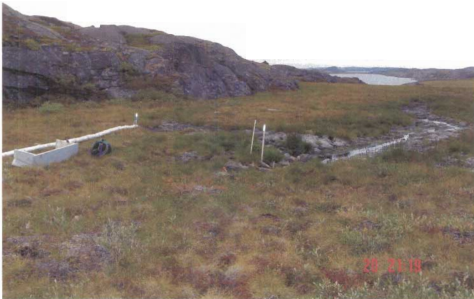
Photo # 5. Sewage system effluent discharge on land behind Windy Camp.
