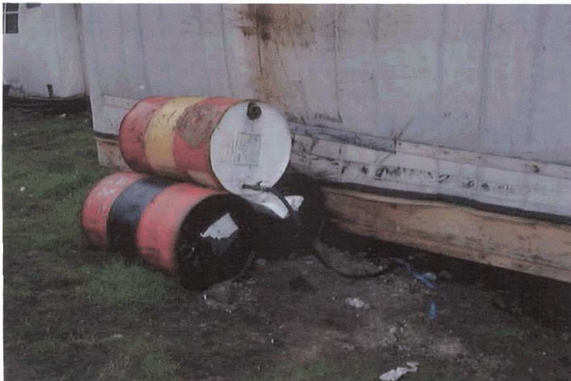
figure 5. Old housing units fuel supply system; 2001/08/12.
