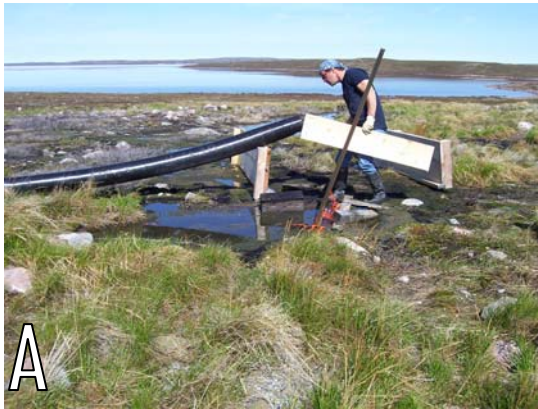
Photographs A & B: Photograph A showing construction of a filter system intended to help reduce the level of total and faecal coliform at the end of the discharge line at Boston camp. Photograph B shows gravel placed in the filter system.
