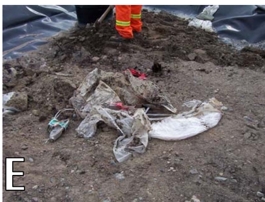
Photographs E & F showing non-biodegradable materials recovered during turning of the contaminated soil stored in the LTA at Boston Camp. Most of these products were plastics and absorbent pads.
