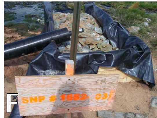
Photographs E & F: Photographs showing the final discharge area. Testing of the system was not possible due to less loading entering into the system.
