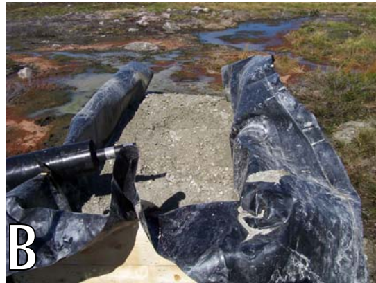
Photographs A & B: Photograph A showing construction of a filter system intended to help reduce the level of total and faecal coliform at the end of the discharge line at Boston camp. Photograph B shows gravel placed in the filter system.
