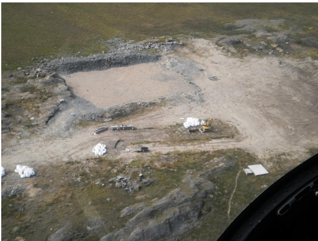
Figure 1. Patch Laydown Contaminated Soil Clean-up Mega Bags Staged for Removal
