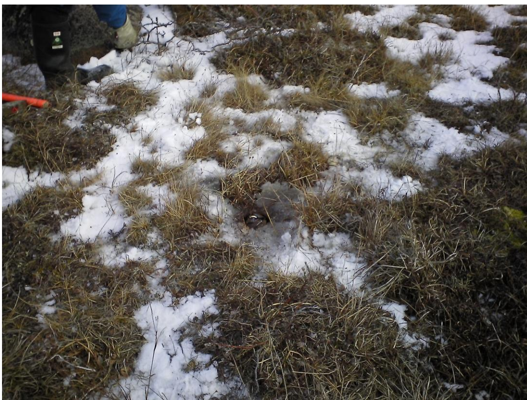
Figure 2. Historical Drill Site Reclamation at hole 07KNK003 with casing cut and hammered closed
