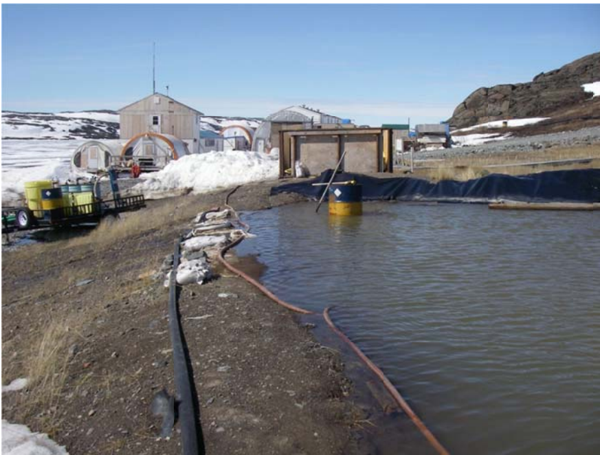
June 13, 2011. Looking north at the low corner of HOP-5 containment facility where the seepage was detected. Note the oil-water separator already in place in preparation for dealing with the water when the pond was thawed.
