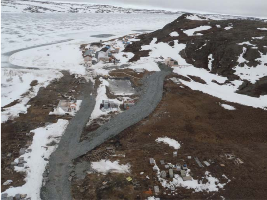
June 4, 2011. Looking north at newly constructed diversion berm and frozen HOP-5 containment facility
