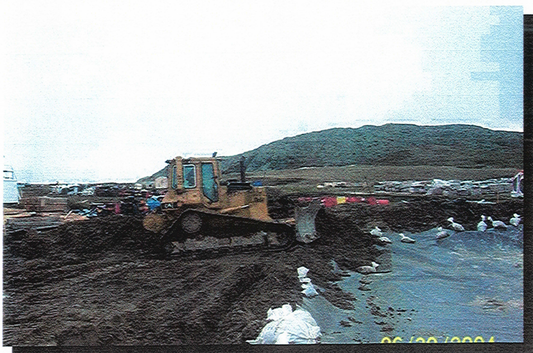
Photo 16 Placement of impacted soil within land treatment area.
