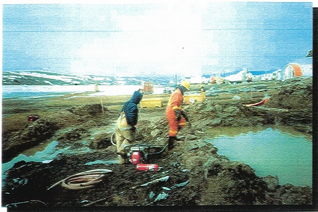
Photo 11 Removal of water within firebreak for treatment and disposal.
