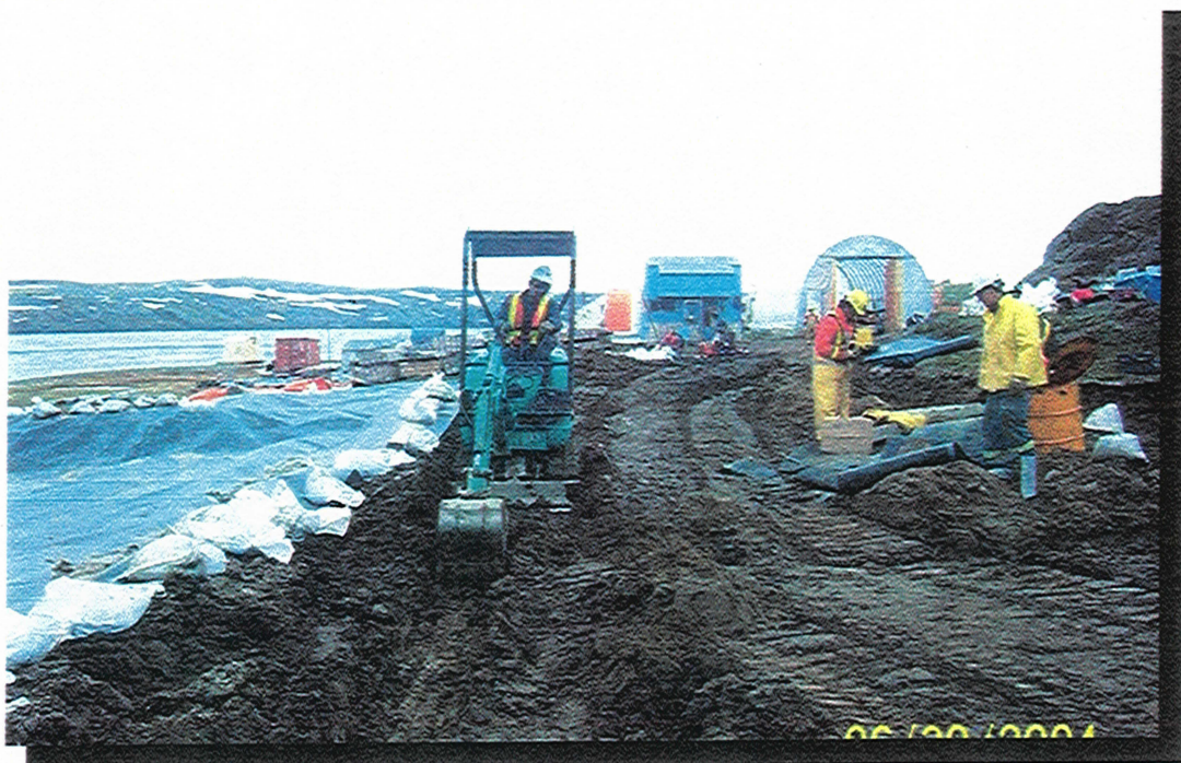
Photo 17 Excavation of drainage trench around land treatment area.
