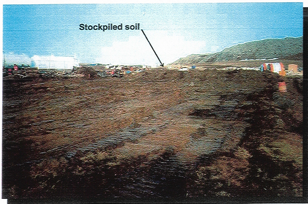
Photo 14 Spill area with impacted soil removed and stockpiled.
