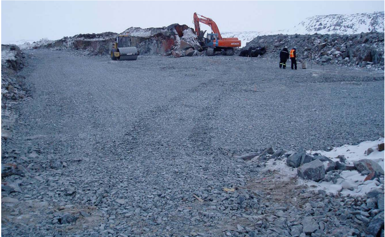
Photo 1: Nearing grade. Excavator pulling out oversize material from daylight area after blast.
