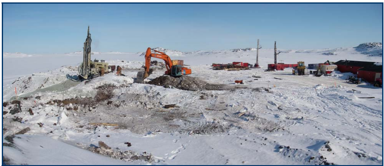
1. Drilling rock on west side; excavator stripping overburden from rock outcrop to be drilled.
