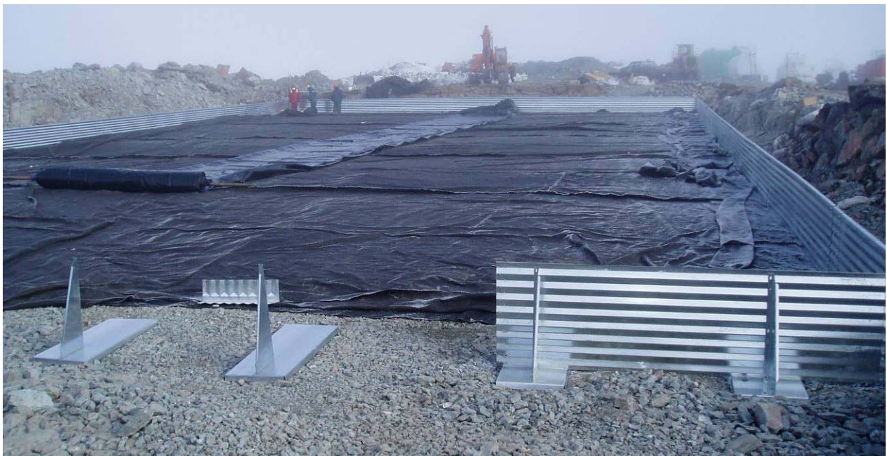
Photo 1: Two layers of geotextile, 80% of the fence, liner is ready to roll out subject to subgrade approval by SRK.
