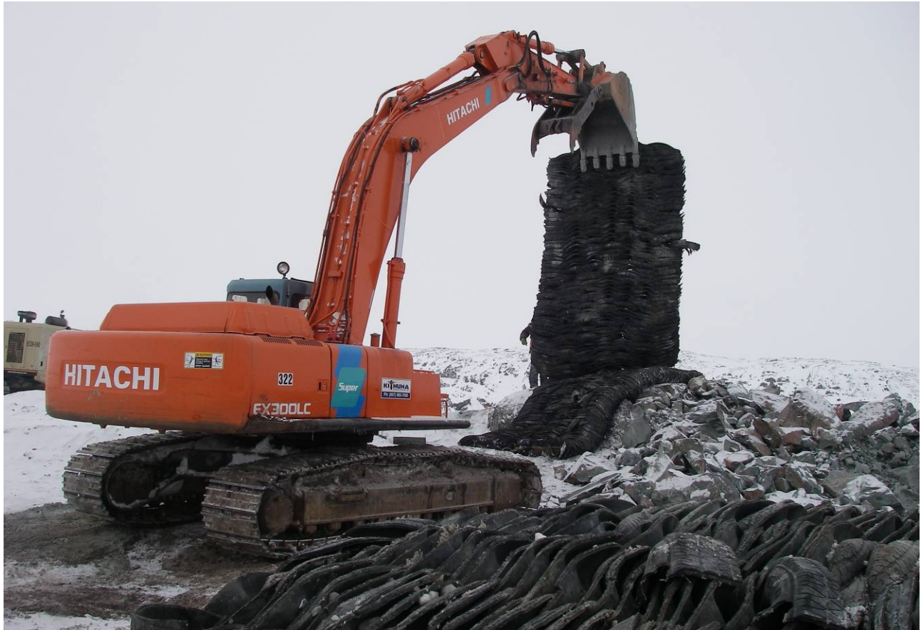
5. Excavator placing blasting mat prior to blast.
