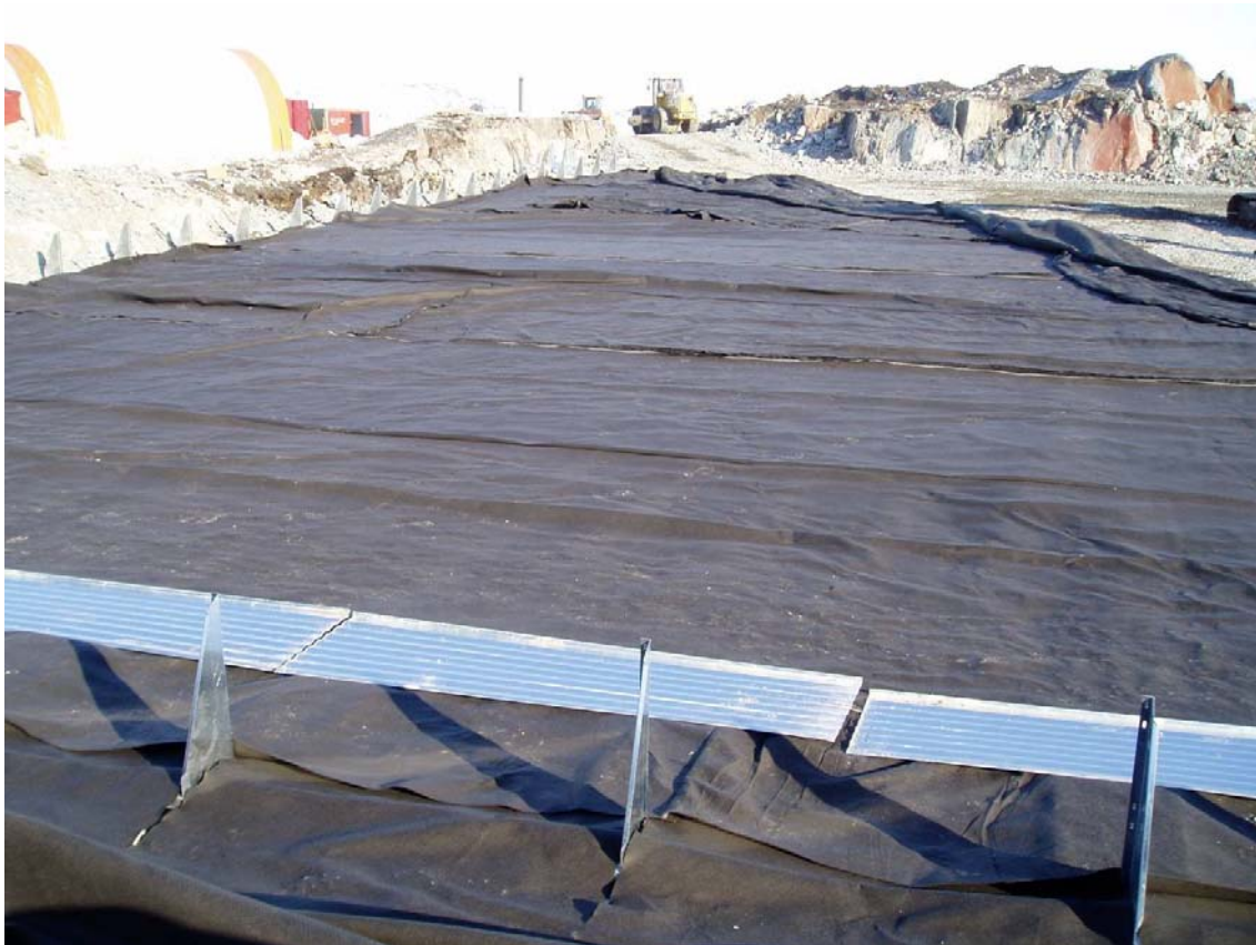
Photo 2: Two layers of geotextile stretched out over floor. Looking south.
