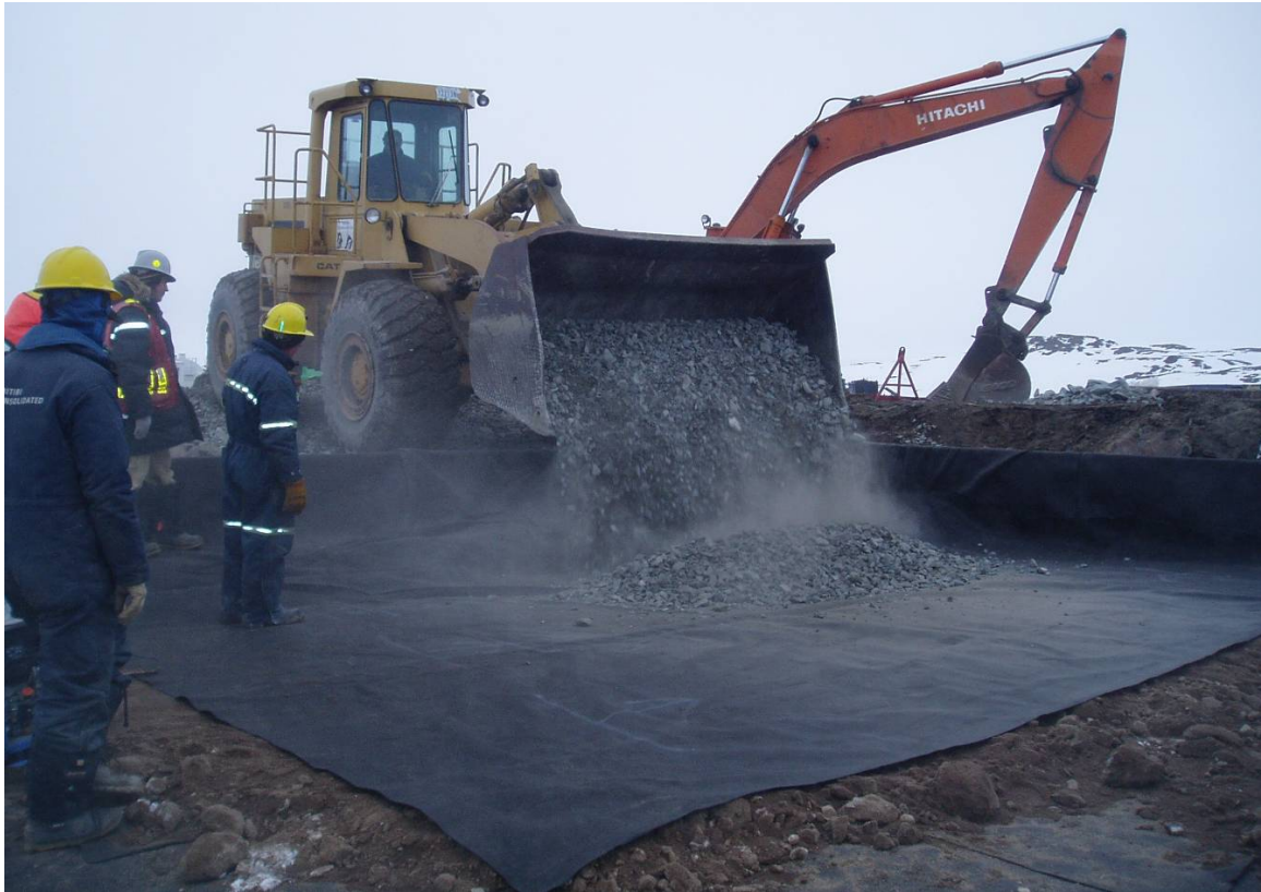
Photo 1: pouring crushed rock over textile, which is over approximately 12 cm of compacted sand.
