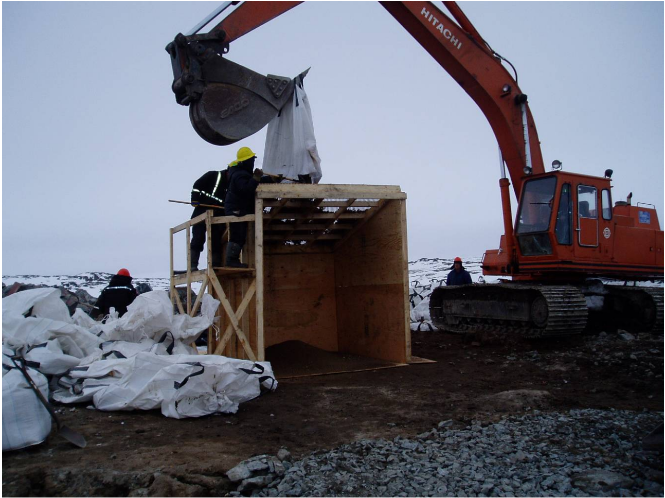
Photo 2: Sand screening operation.
