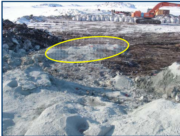
2. Completed drill holes in foreground; outline indicates high area of rock to be trimmed.
