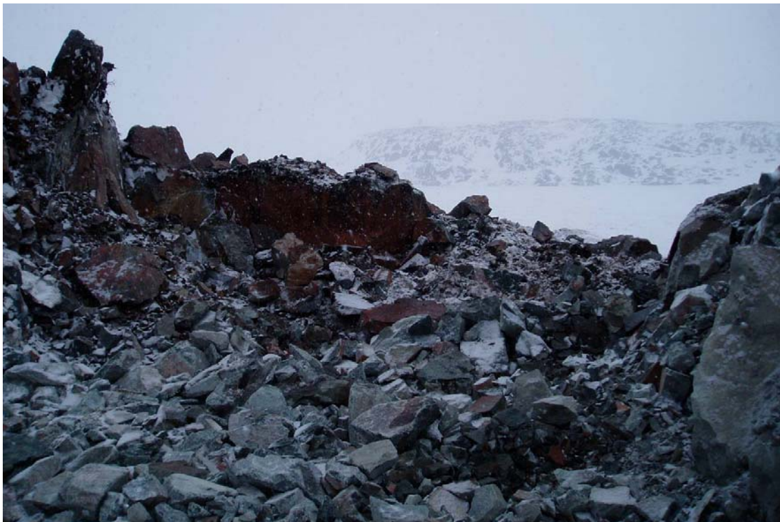
Photo 2: Rock wall at daylight point which needs to be removed.
