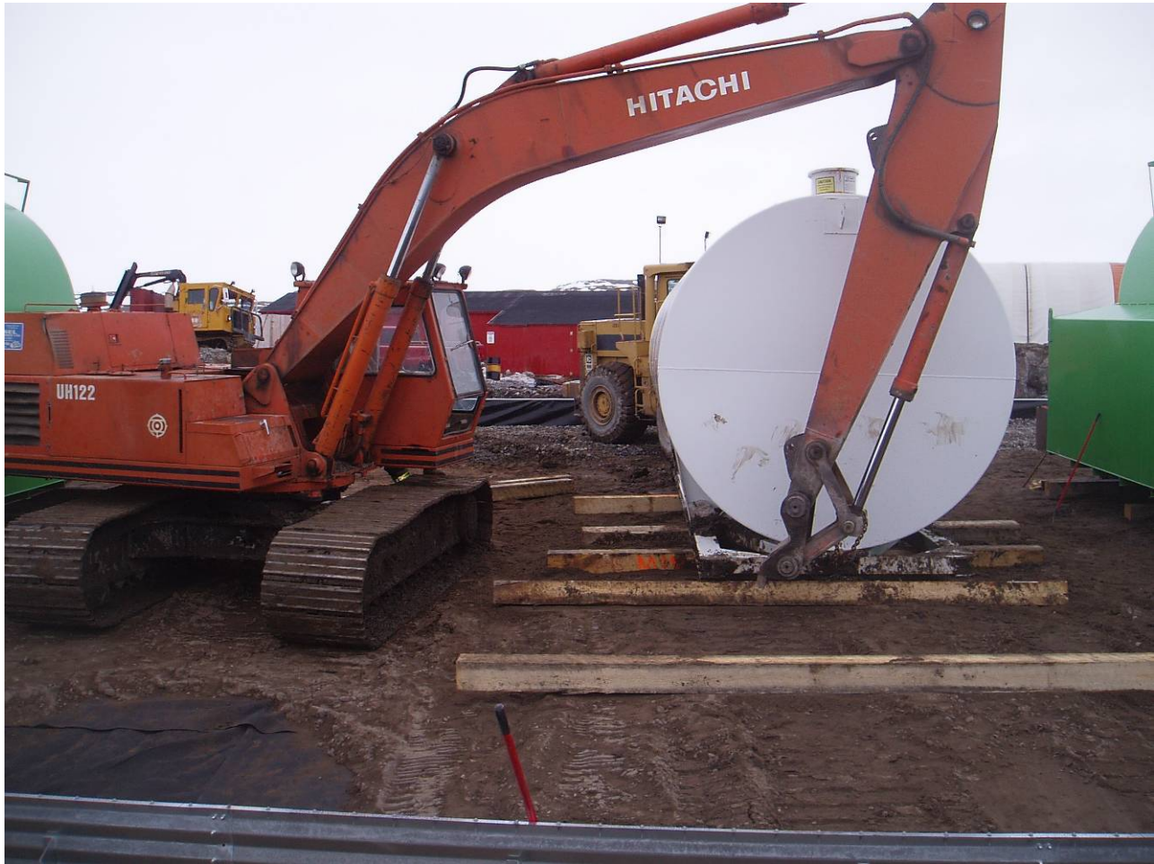
Photo 1: Movement of the last tank into place.
