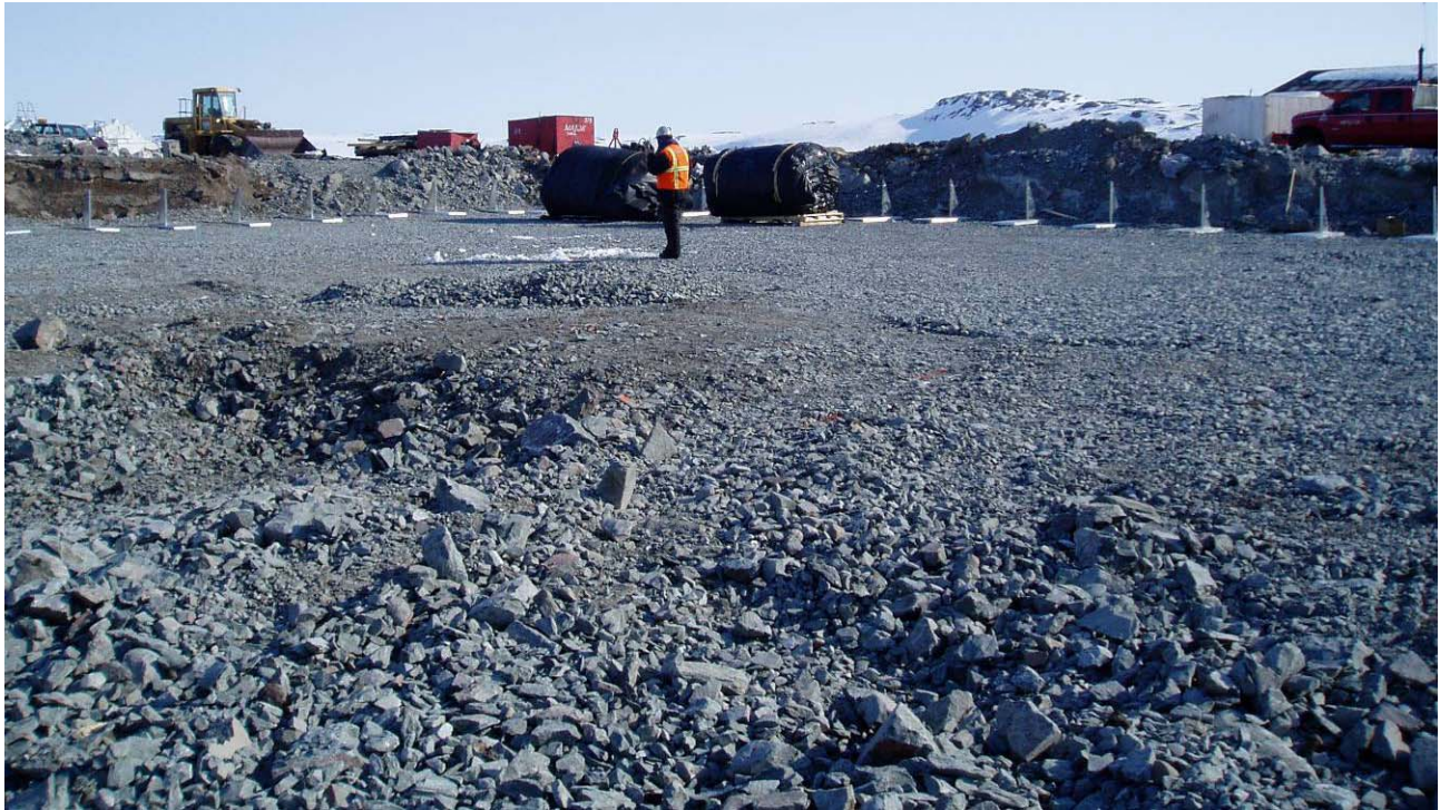
Photo 1: North and East walls of Tank Farm, with fins and base plates in place. Sump in foreground.
