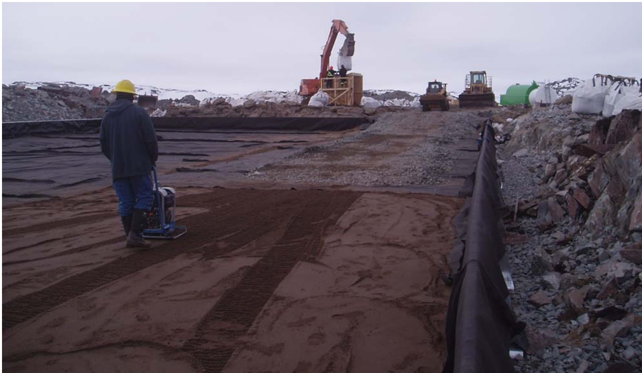
Photo 1: View looking north of sand material being screened, and construction of the road across the tank farm.
