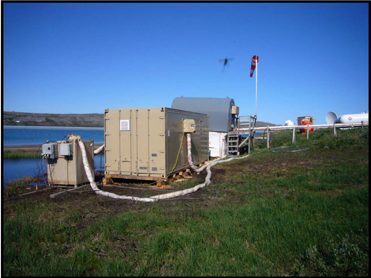
Figure 3-5: Photograph of the Two RBC units at the Windy Lake Camp
