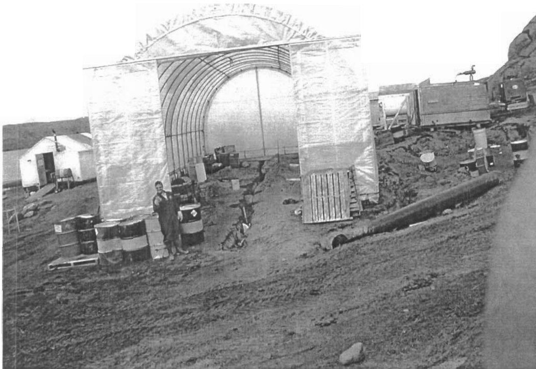
Photo #5: Trench and test holes in storage shed.
