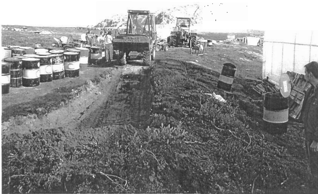
Photo #3: Kabota excavating contaminated soil.
