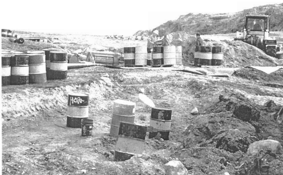
Photo #4: Transferring contaminated soil into 45 gallon drums.
