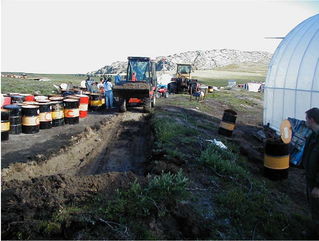
Photo #3: Kabota excavating contaminated soil.
