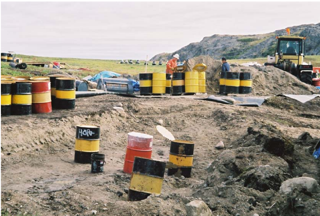
Photo #4: Transferring contaminated soil into 45 gallon drums.
