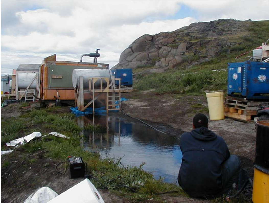
Photo #1: Generator tank and spill ponded behind natural berm.
