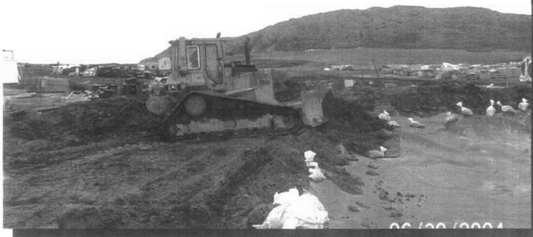
Photo 16 Placement of impacted soil within land treatment area.
