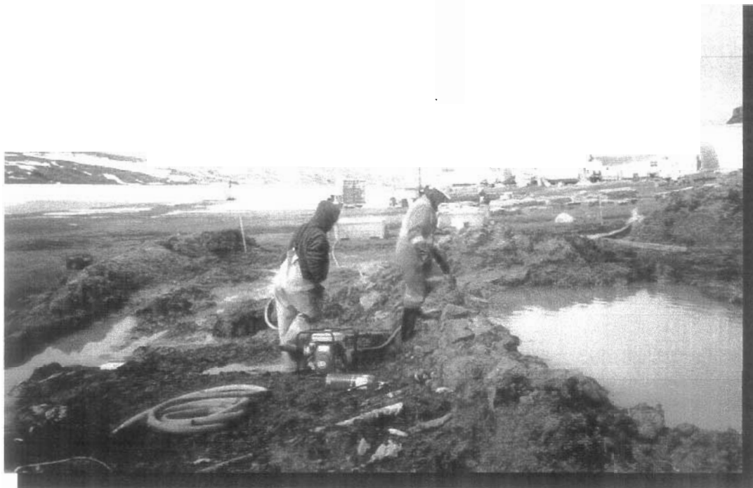
Photo 11 Removal of water within firebreak for treatment and disposal.
