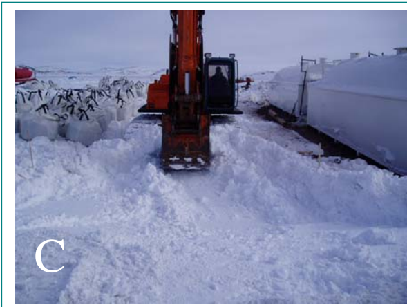
Photograph C: Removing snow with a backhoe. Photograph D: Spreading sand on the next pad before pulling a tank.
