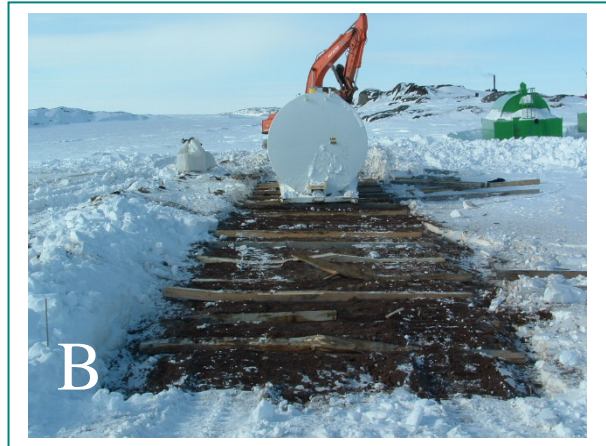
Photograph A: Preparing first sand pad. Photograph B: First AST tank (50,000 L) placed on the pad within the farm.
