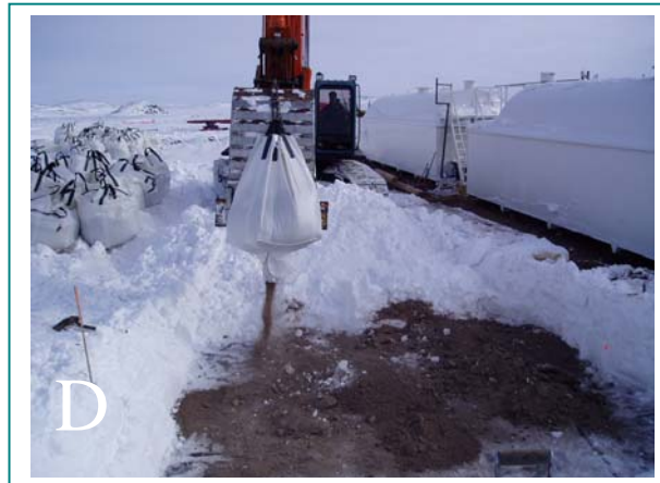
Photograph C: Removing snow with a backhoe. Photograph D: Spreading sand on the next pad before pulling a tank.
