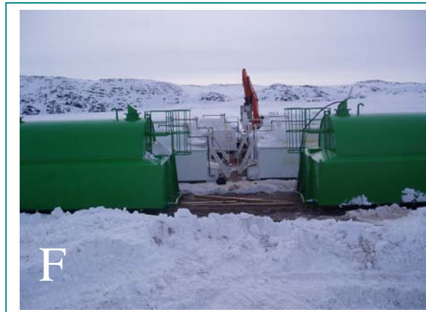
Photograph E: Pulling a 70,000 L AST tank onto the pad. Photograph F: All (8) AST tank placed onto the pads within the farm.
