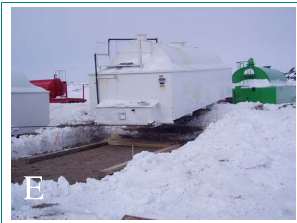
Photograph E: Pulling a 70,000 L AST tank onto the pad. Photograph F: All (8) AST tank placed onto the pads within the farm.
