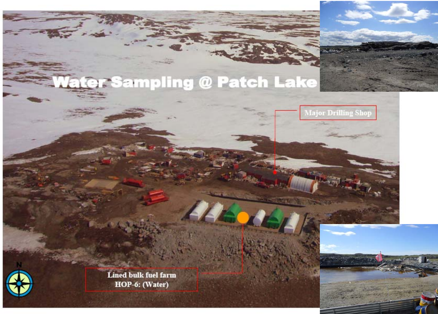
Figure B2 Patch Lake Fuel Farm – Prior to Decommissioning in 2009/2010.
