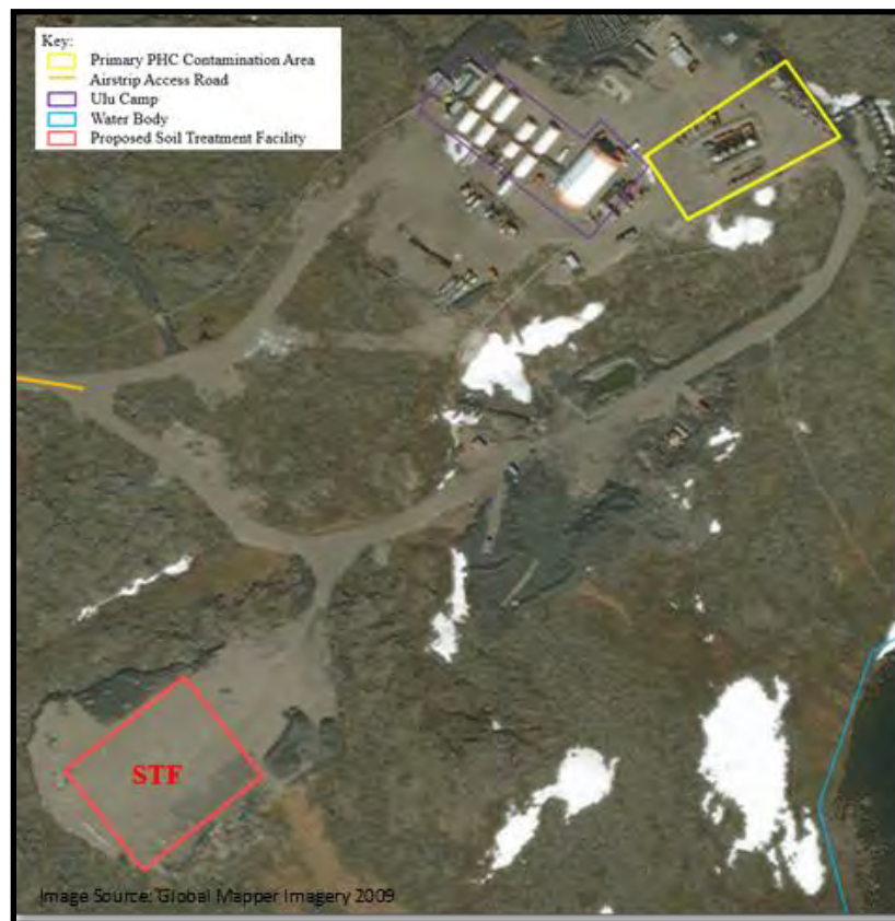
Figure 9. Soil treatment facility overview
