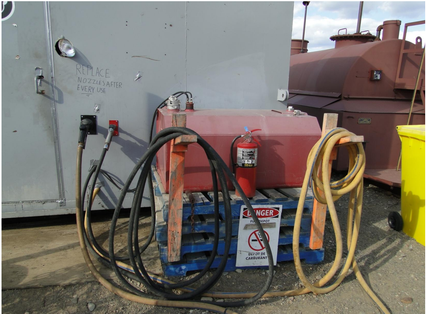
Figure 4. Fuel Transfer Station. Nozzles contained to avoid drips; spill kit visible.
