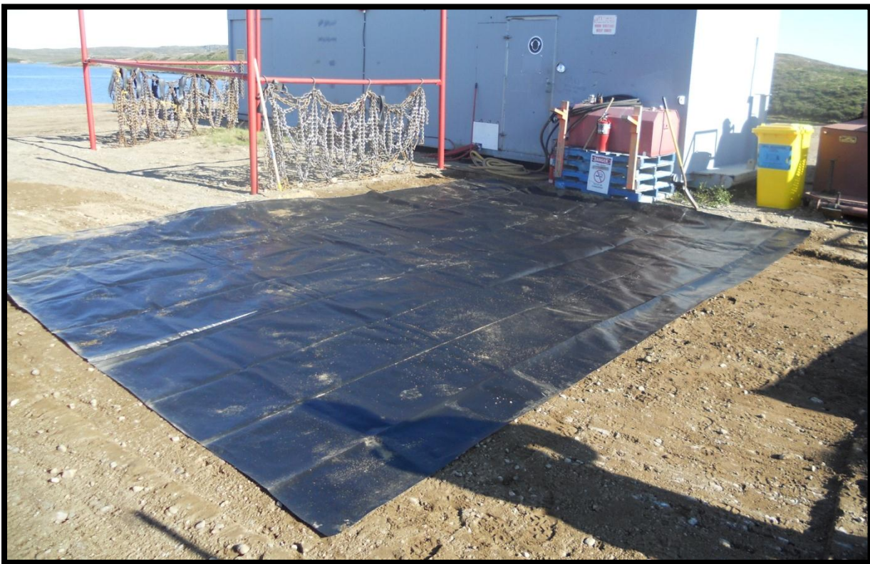
Photo 2: Liner before being buried.
