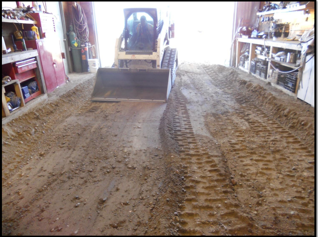
Photo 4: Shop floor being excavated for liner installation.
