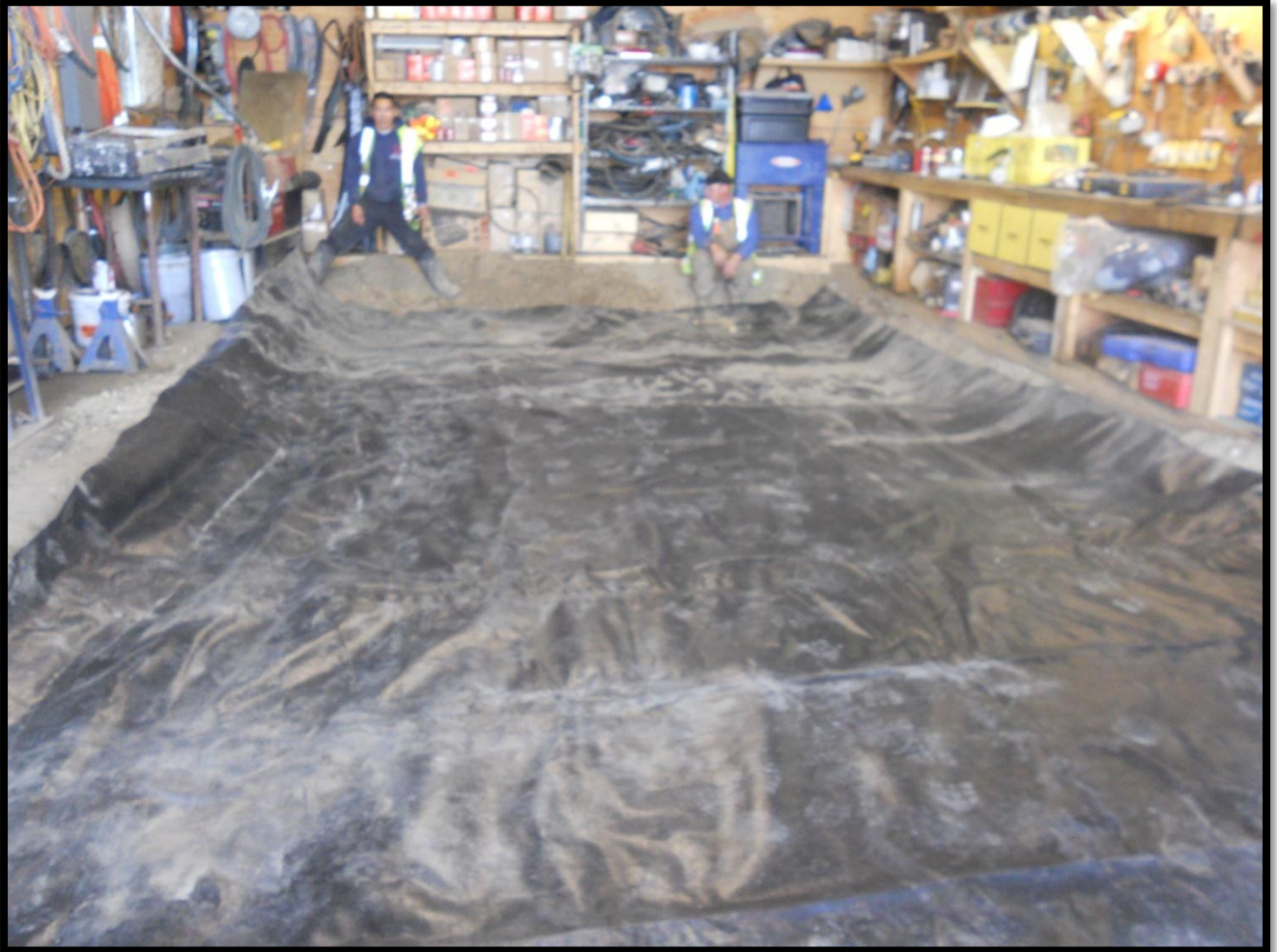
Photo 6: Liner before being backfilled.
