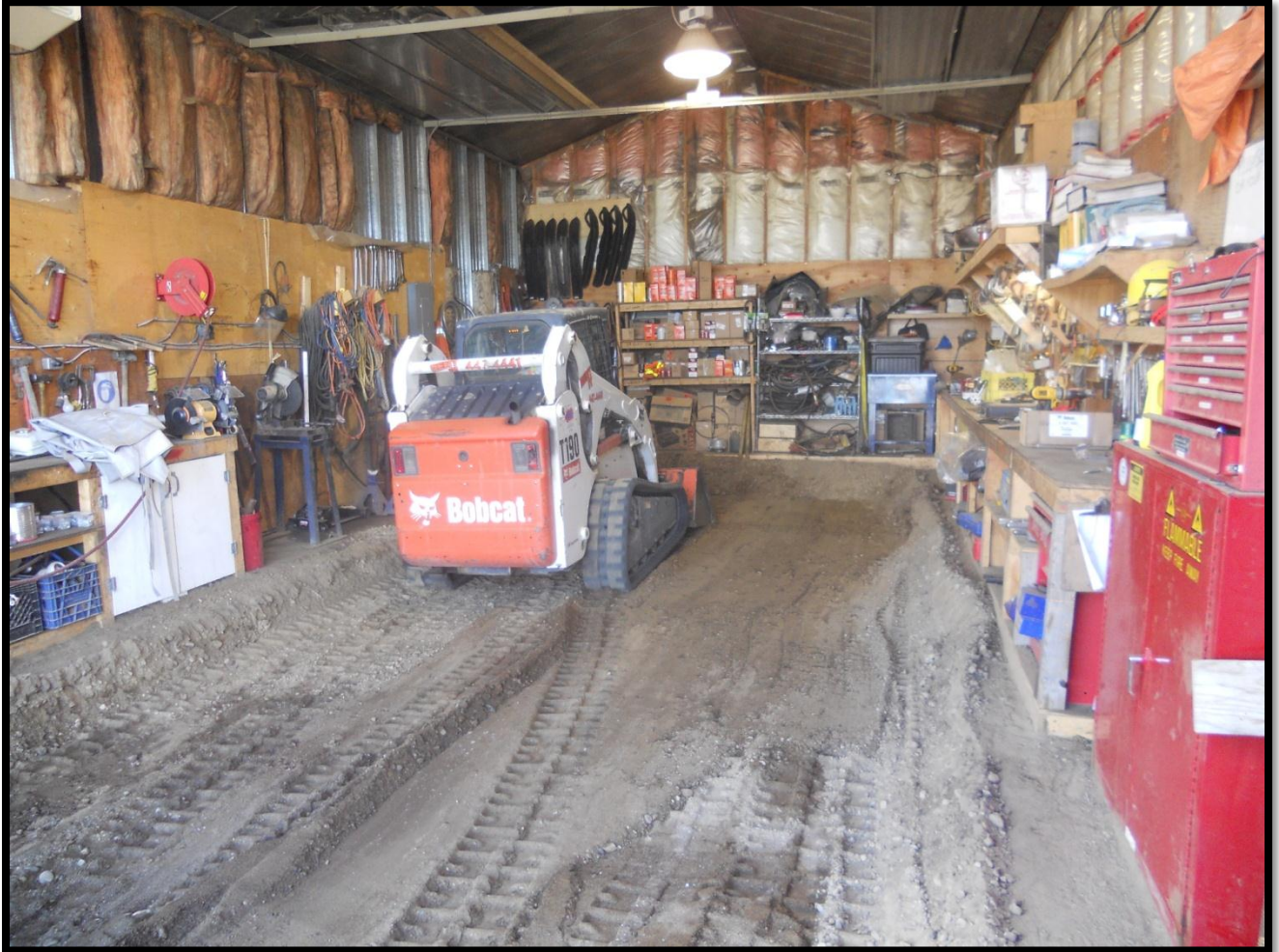
Photo 5: Shop being excavated for liner installation.
