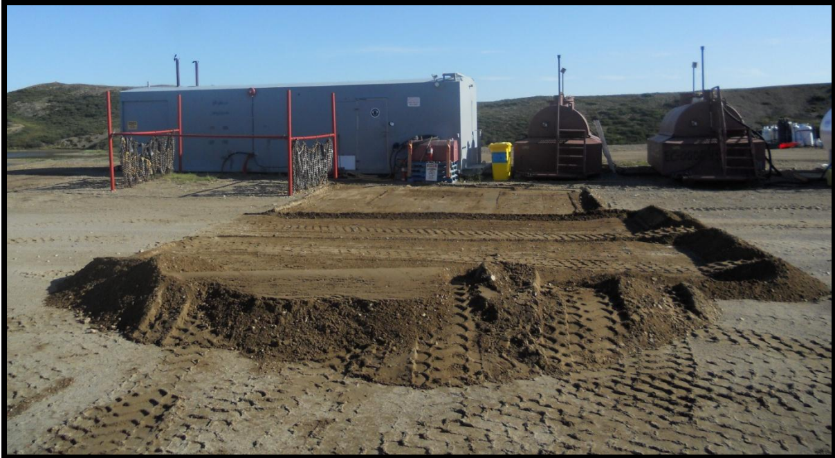
Photo 1: Area excavated for liner.
