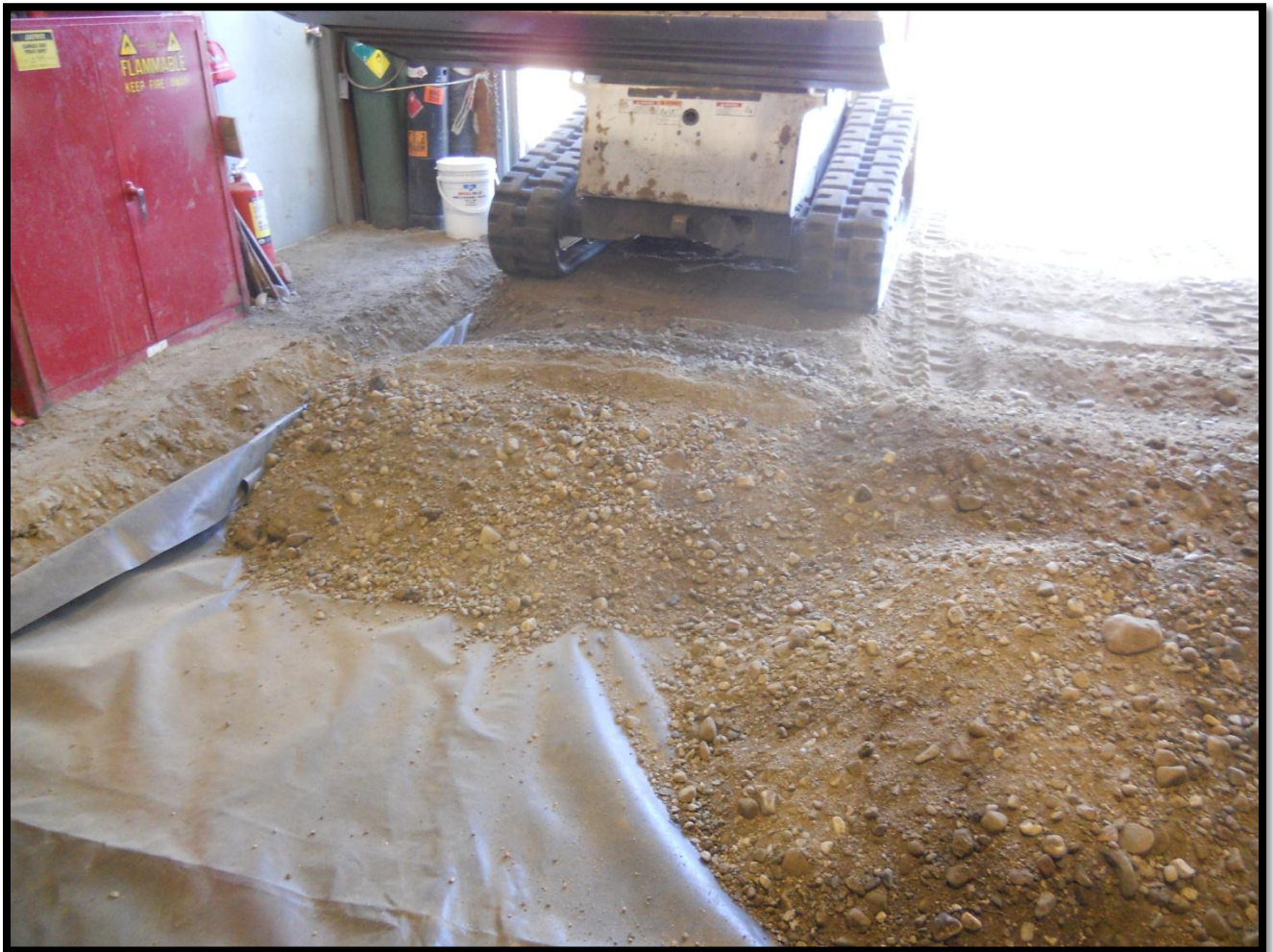
Photo 7: Shop liner being back filled.
