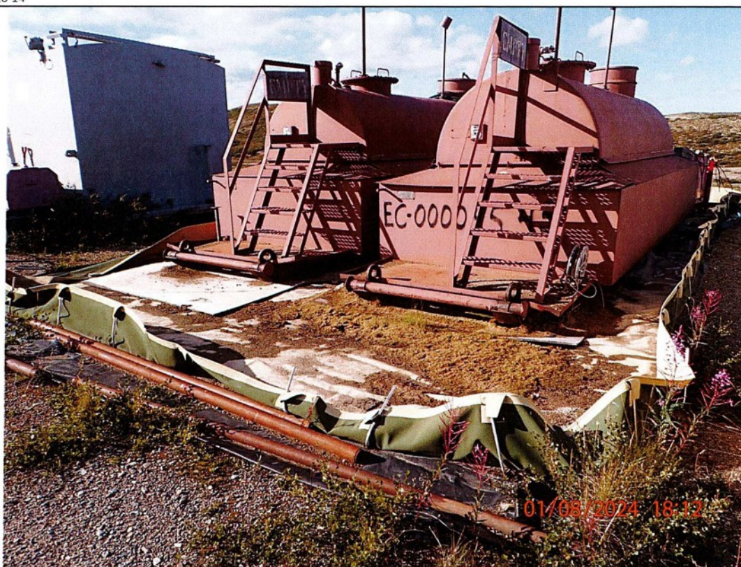
Failed secondary containment. Moss and some water present inside the berm.
