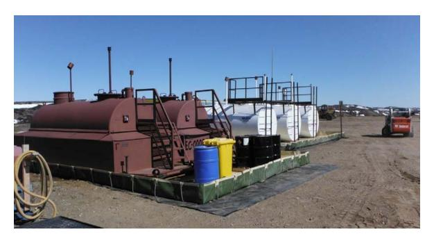
Fuel farm after installation of secondary containment berms
