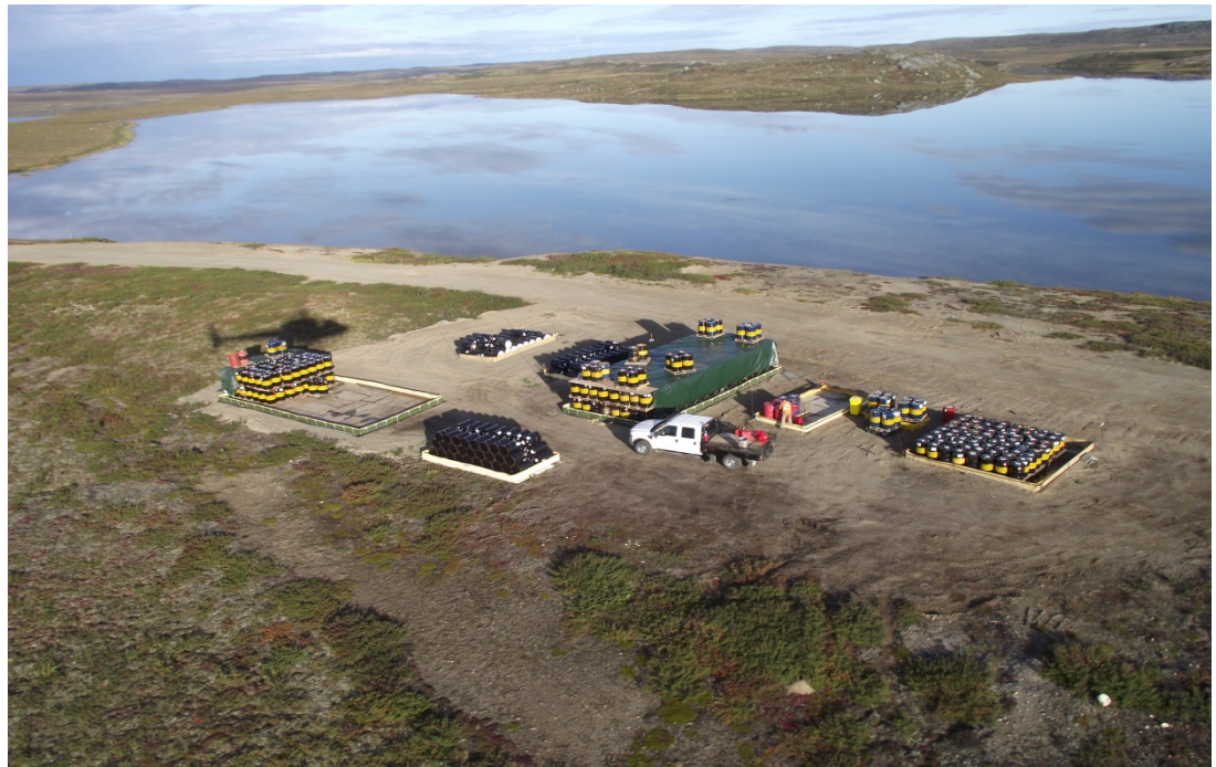
Drum storage onsite with secondary containment berms – August 2012
