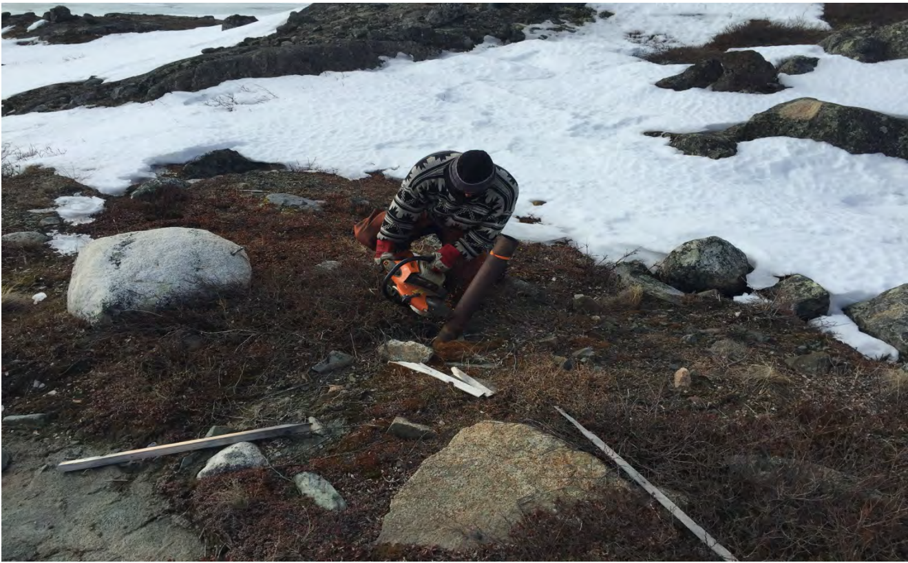
Cutting and capping historic drill casings at ground level
