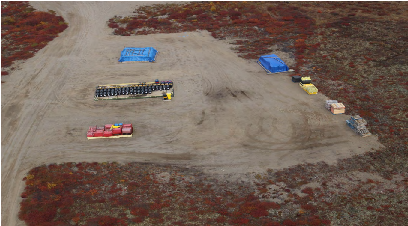
Drum fuel storage area at end of 2014 season. All of this has now been removed from site.
