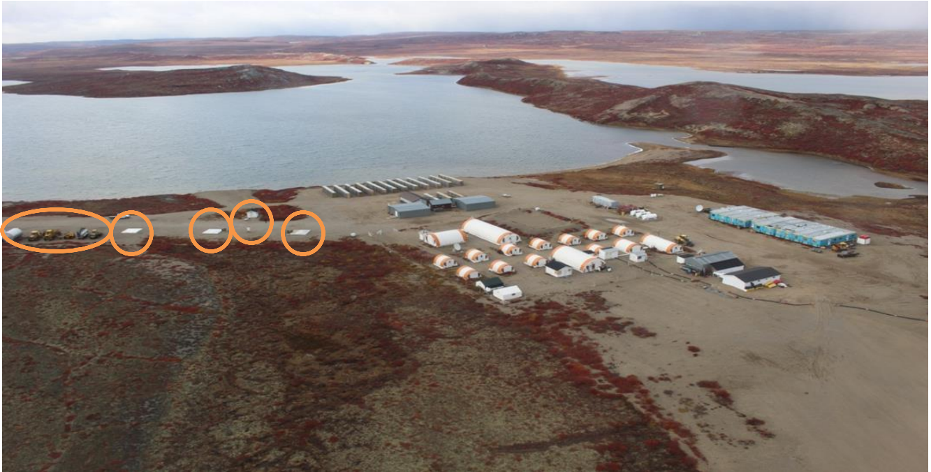
Izok (Ham Lake) site. The equipment and structures indicated by the orange circles were removed in 2015. Photo – July 2015
