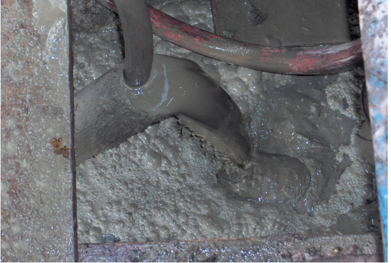
Photo 12 - Cementing Drill Hole at Lucky 7
