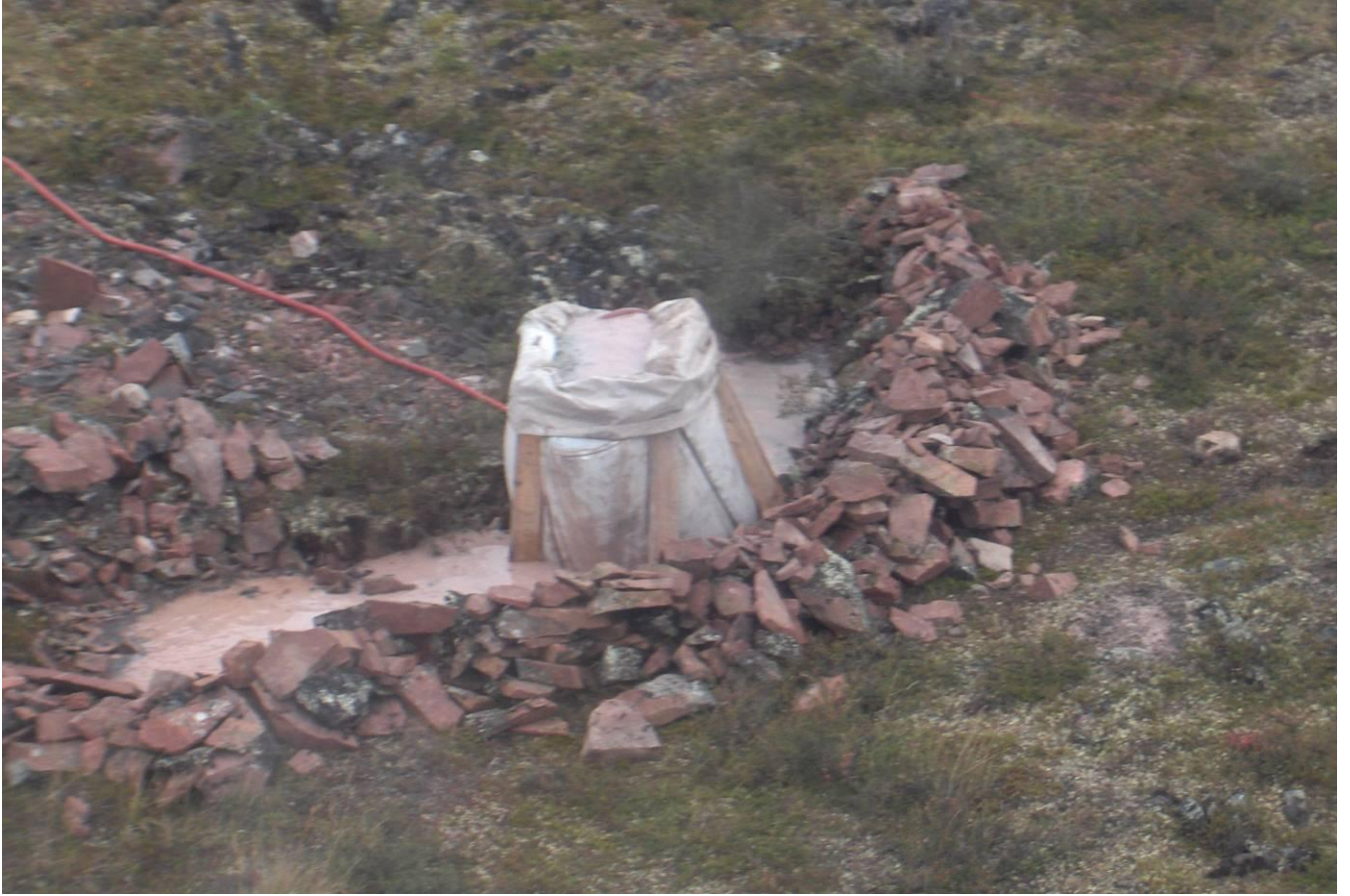
Photo 23 - KZ Zone - Large Bag Catches Rock Cuttings in Sump
