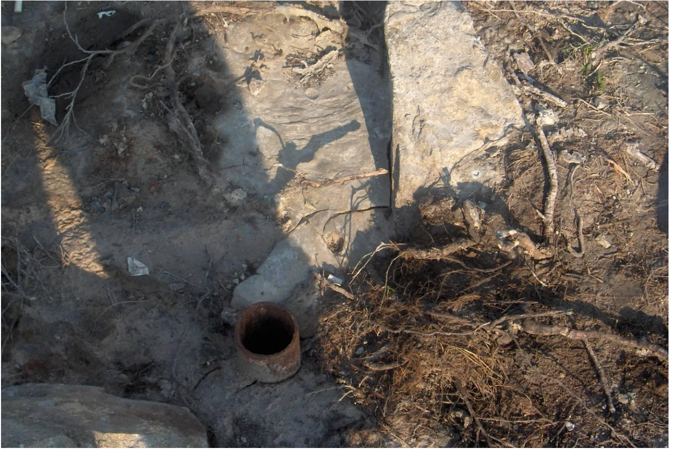
Photo 18 - KZ Drill Hole KZ-07-07 Cemented Hole and Anchor Cut near Ground Level
