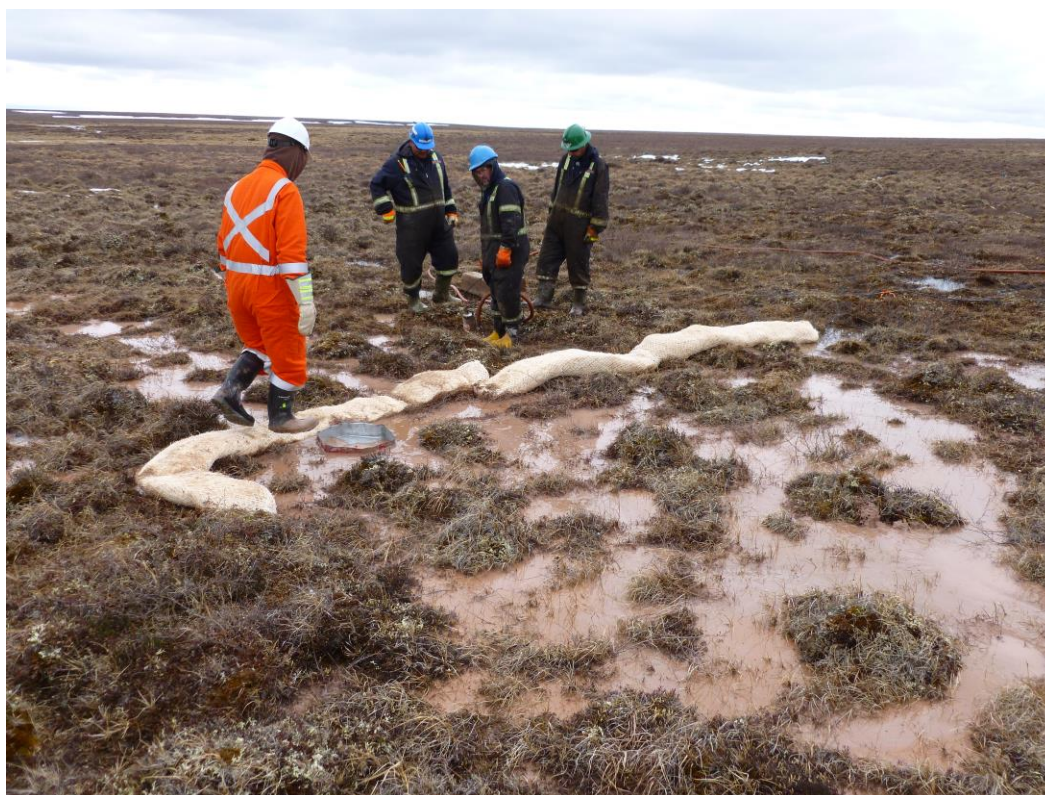
Photograph 4. Containing the Spill on June 17, 2015
