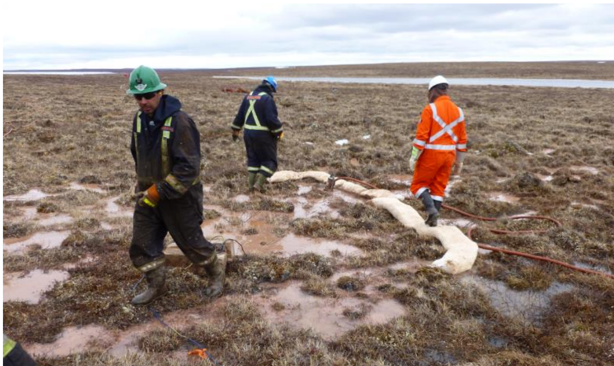
Figure 4. Installation of Filter Socks and Sump Pump on June 17, 2015
